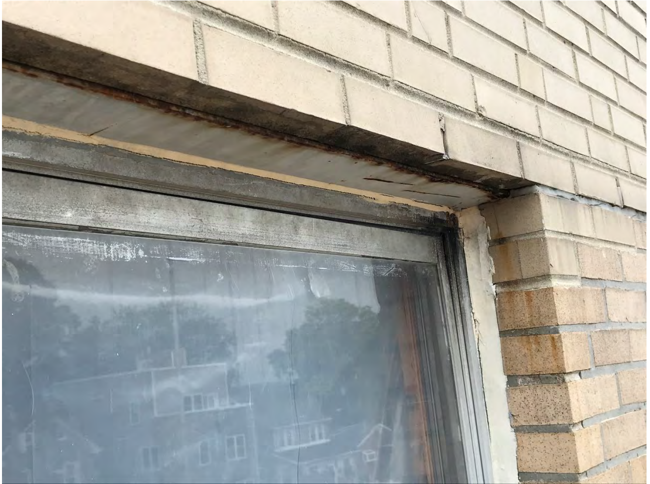
(North Wall Lintel)
