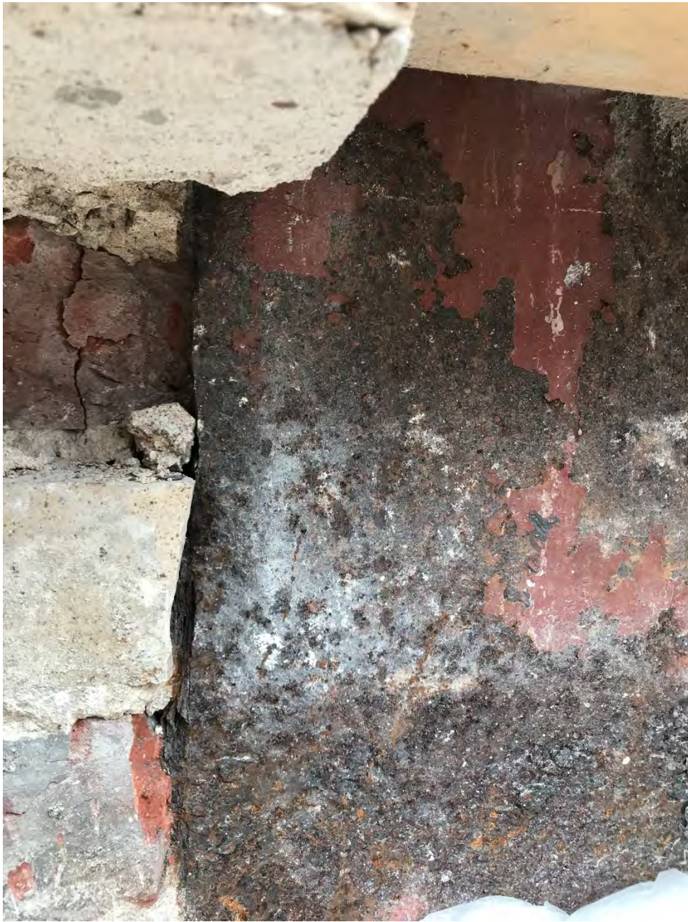
(West Wall Column)
