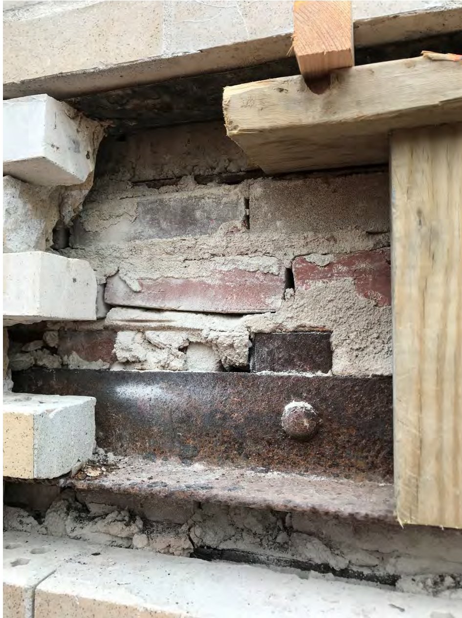
(North Wall Shelf Angle)
