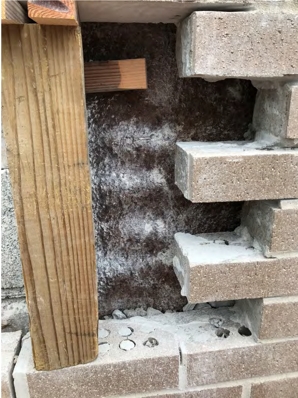
(West Wall Column)
