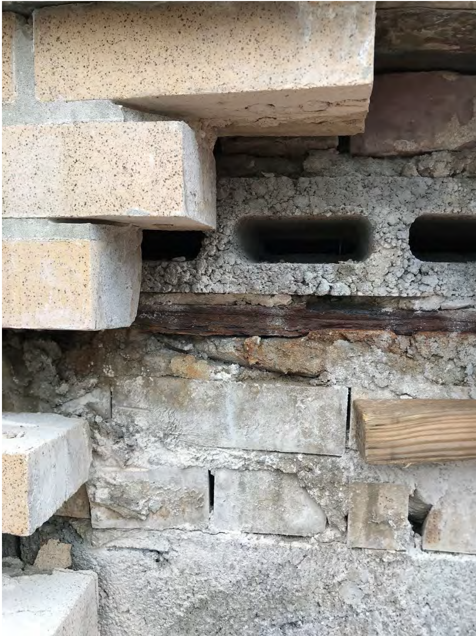
(West Wall Roof Beam)
