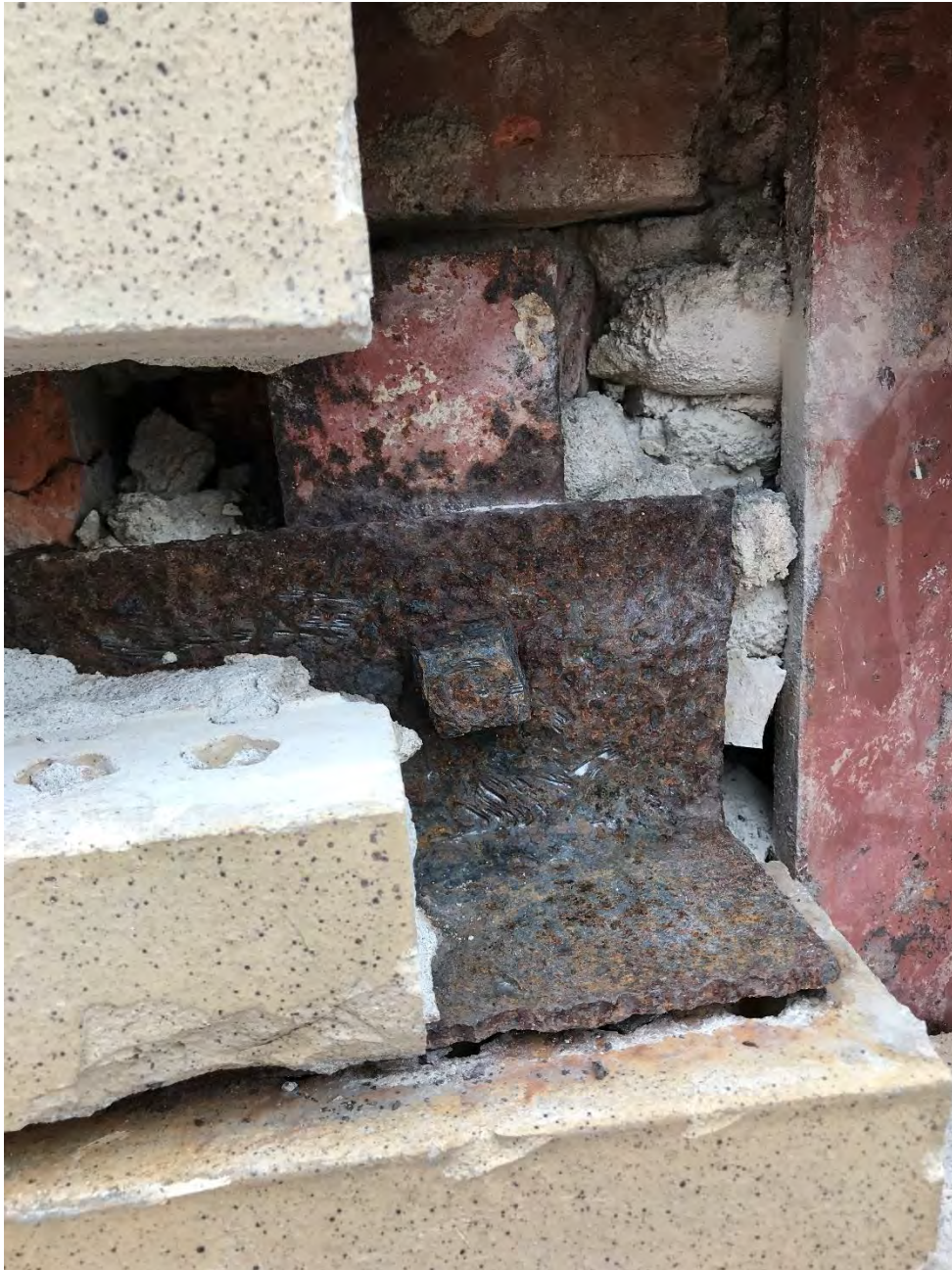
(North Wall Shelf Angle)
