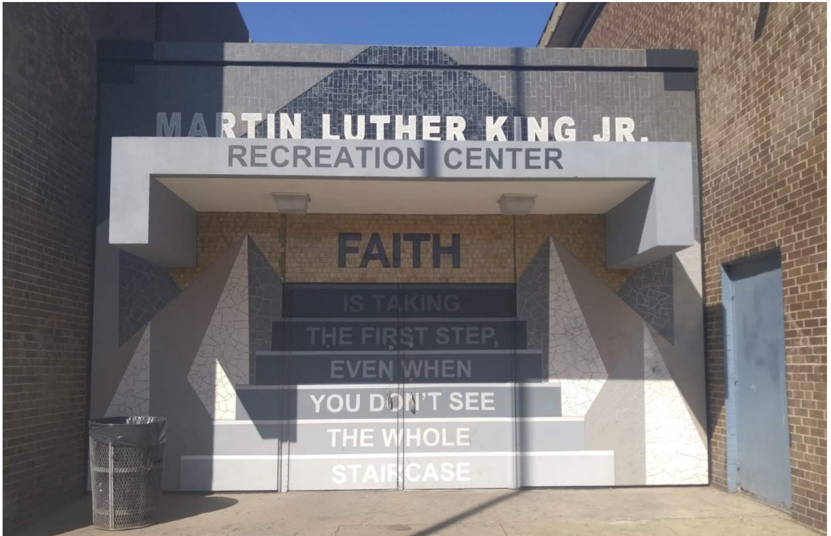
Front Entry Canopy - Area 9
