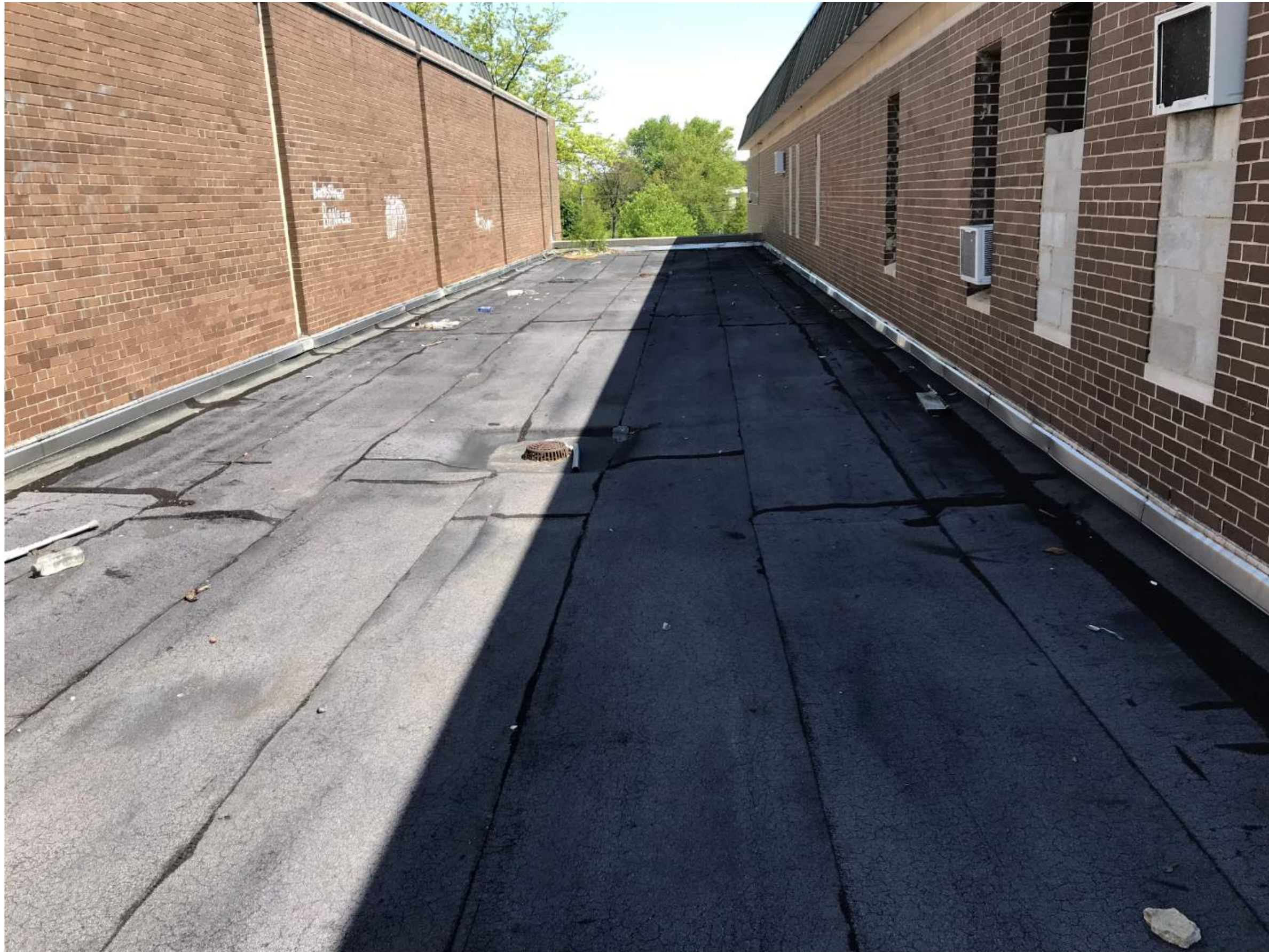
Corridor Link Roof - Area 2
