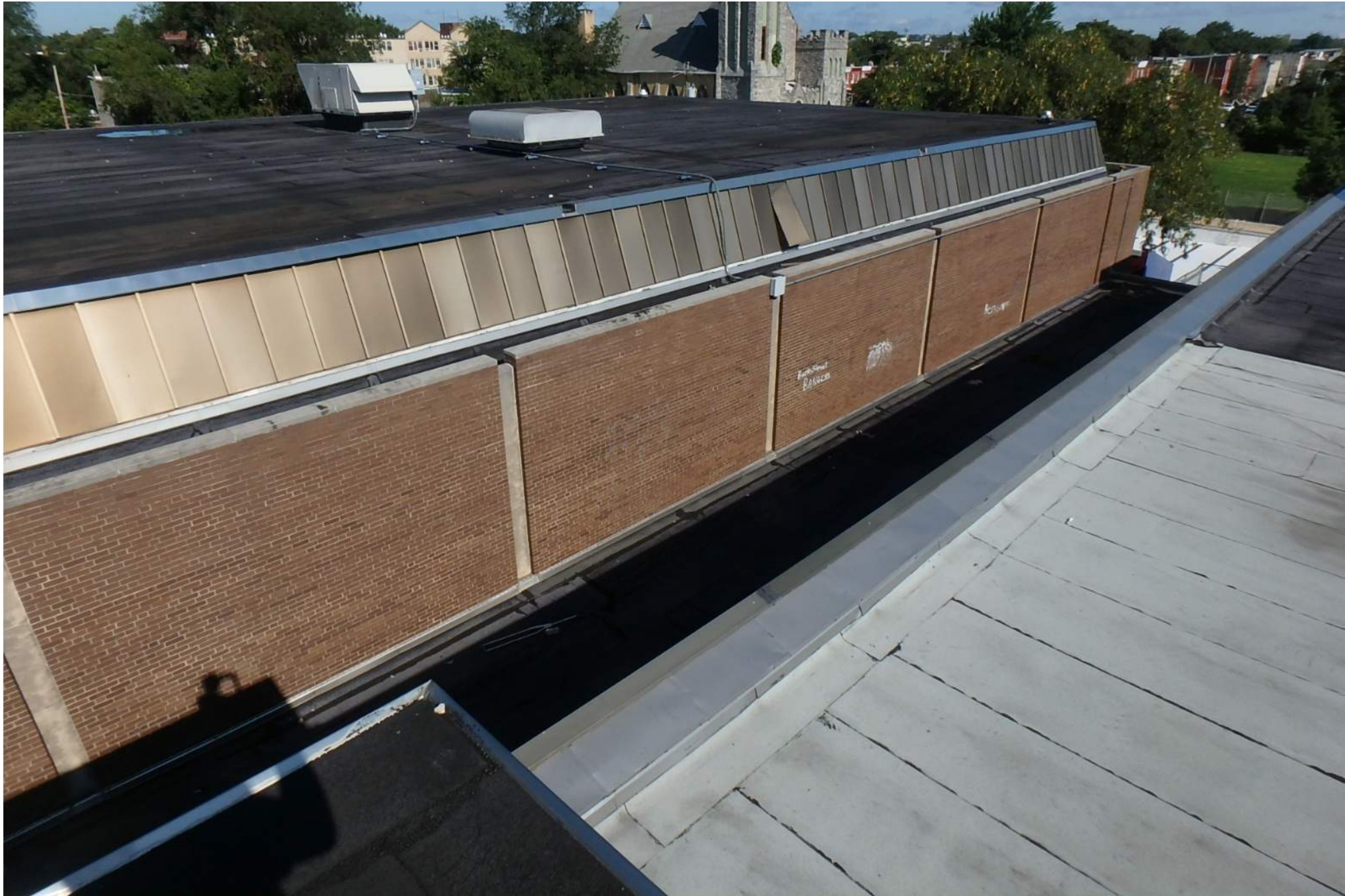
Corridor Link @ Area 1A - 3A Roof
