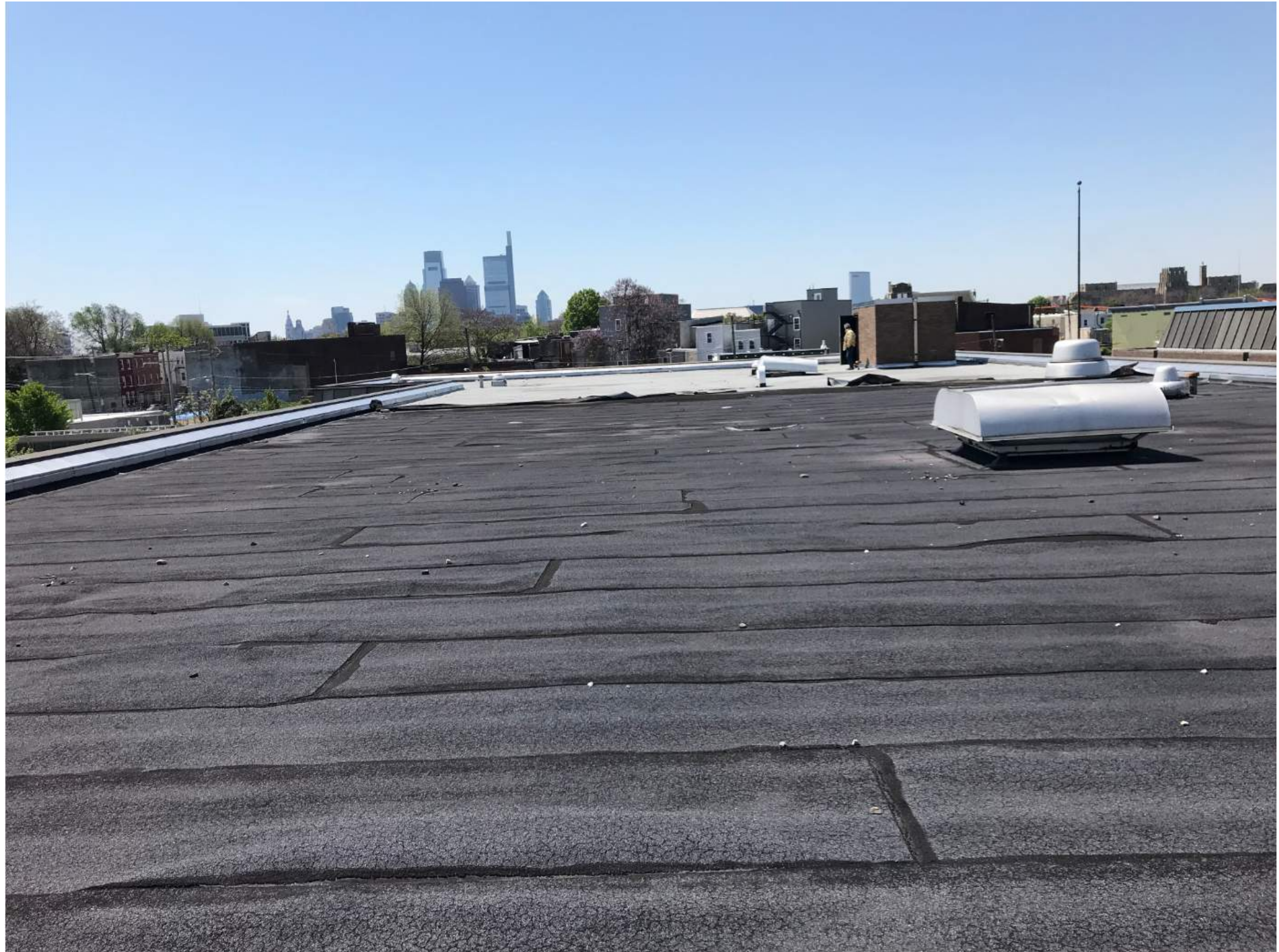
Rec Center - Area 3A Roof (1)
