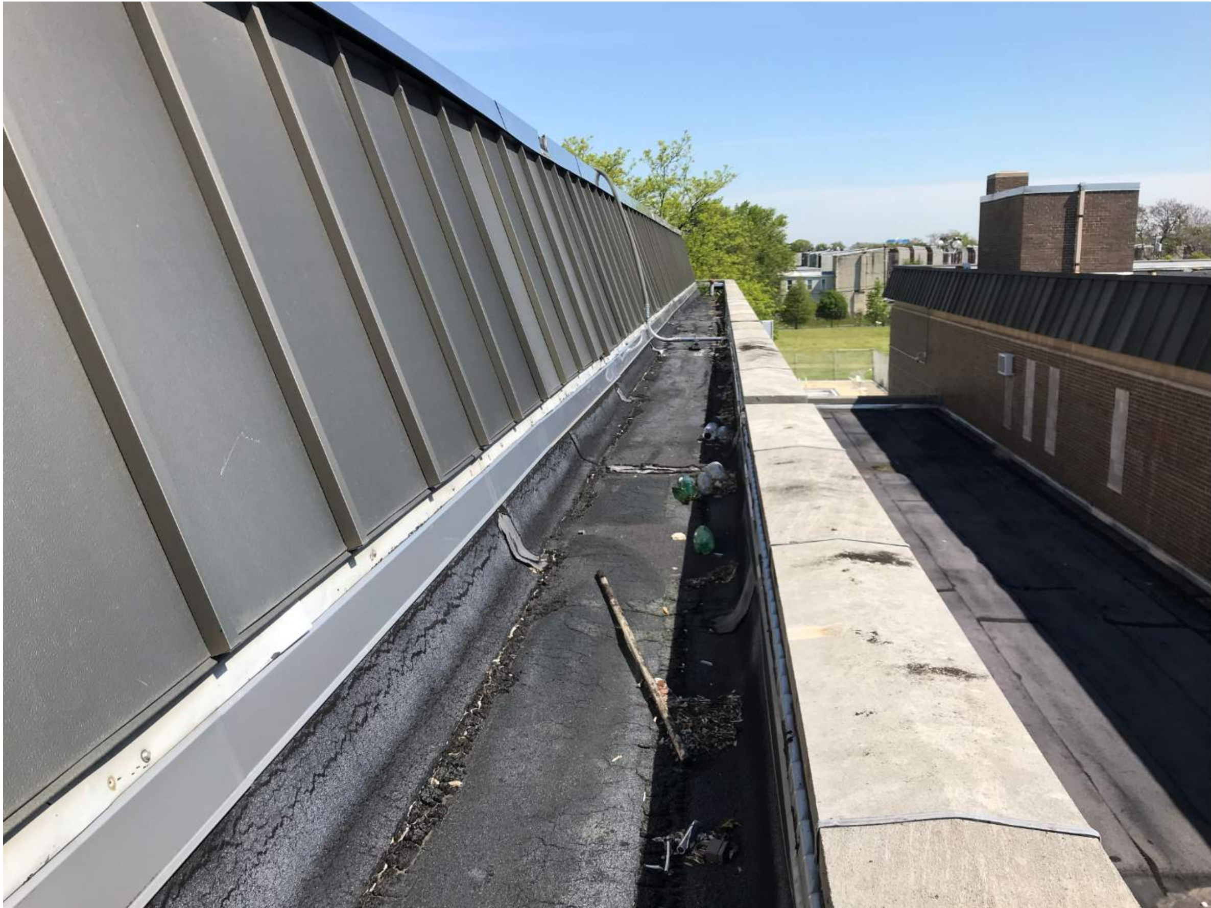
Gym Roof - Area 1B Gutter & 1C Mansard
