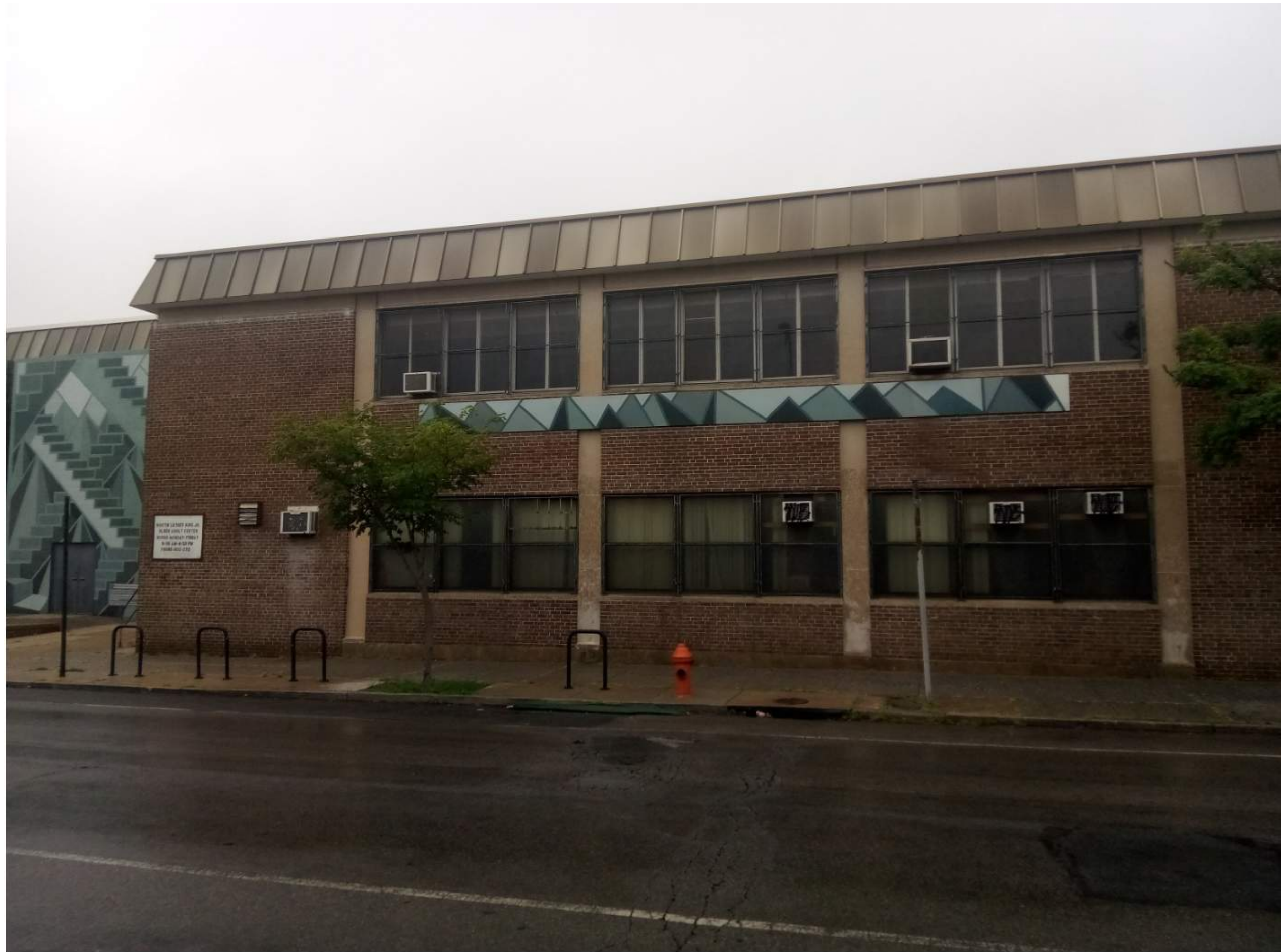
Rec Center - Area 3B Mansard Roof
