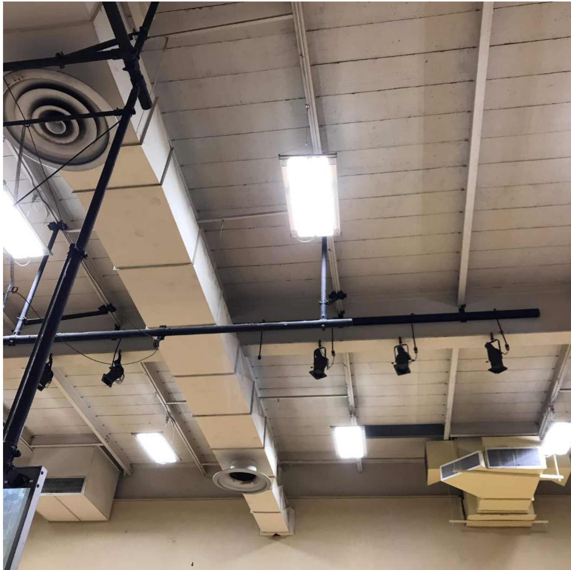
Gym Structure @ Area 1A Roof
