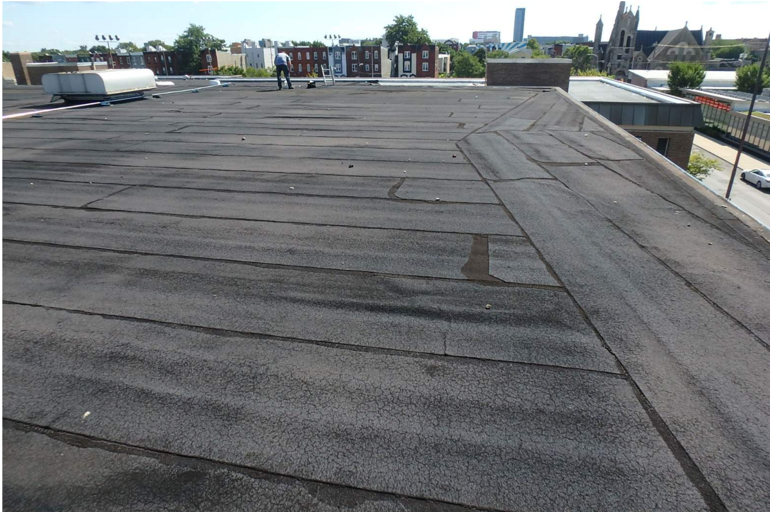
Gym - Area 1A Roof
