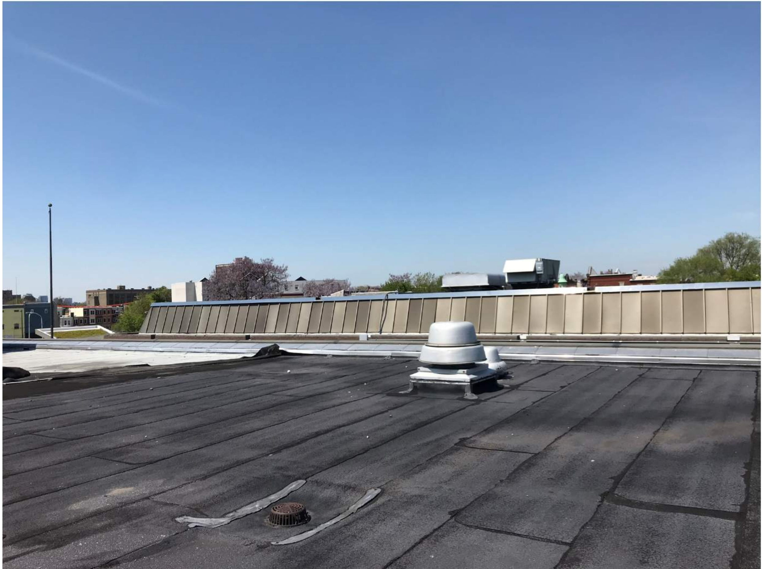
Rec Center - Area 3A Roof (2)
