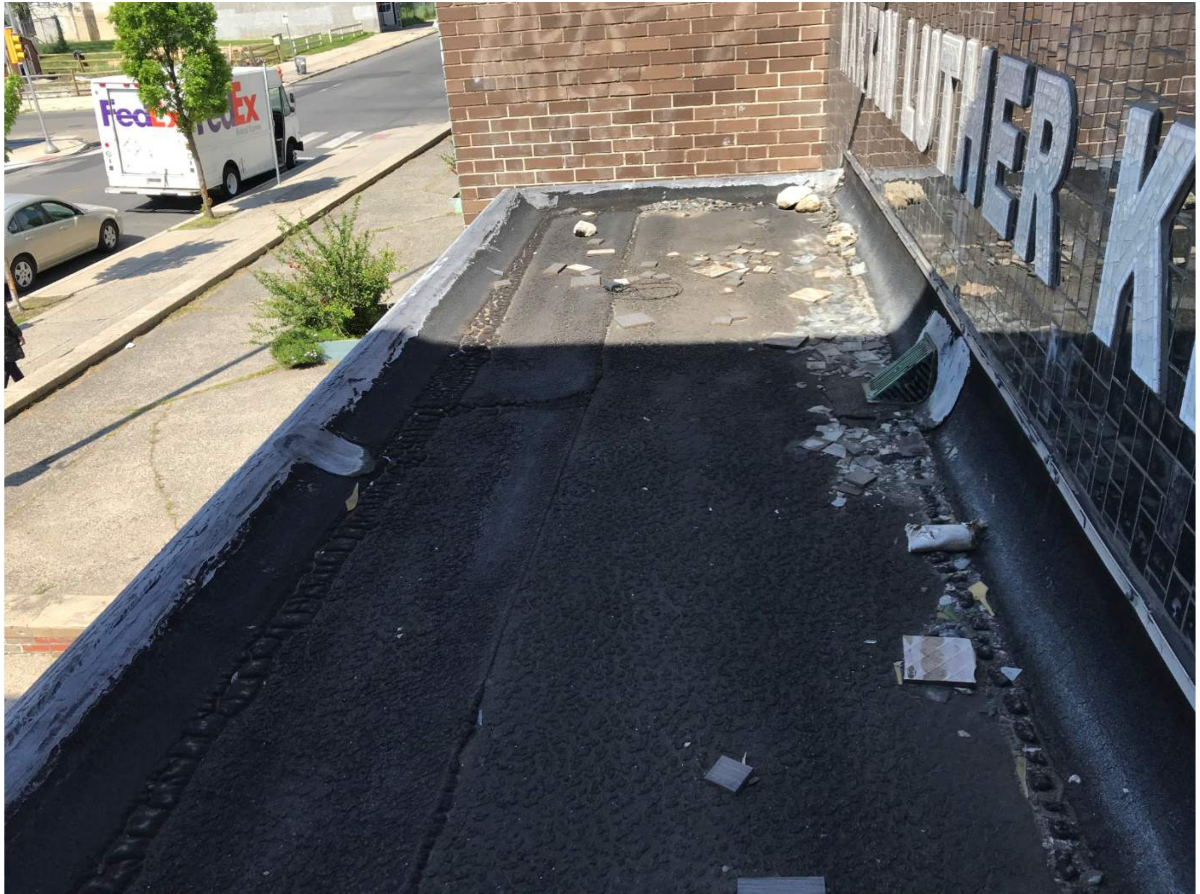
Front Entry Canopy Roof - Area 9
