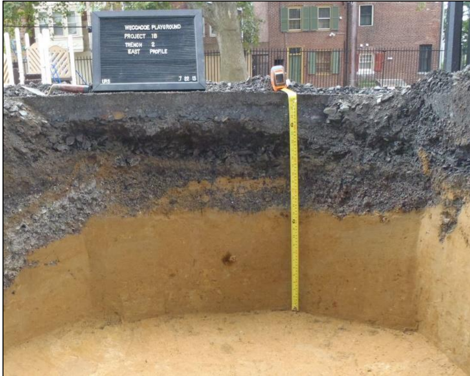
Figure 2. Asphalt and gravel sub-base exposed in the Trench 2 east profile (URS 2013).
