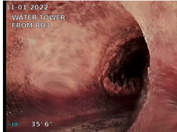
14, 00:02:26, 35.50ft Miscellaneous General Observation / WYE RIGHT
