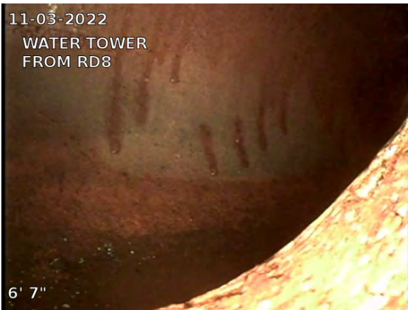
7, 00:00:50, 6.58ft Tee Connection / TIES INTO MAIN
