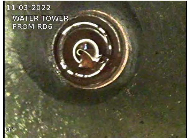
2, 00:00:00, 0.00ft Water Level, 100% of the vertical dimension / TRAP AT BOTTOM OF RISER
