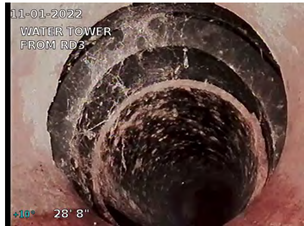
12, 00:02:01, 28.67ft Miscellaneous Material Change, Cast iron / CHANGE TO CIP
