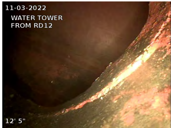
8, 00:00:47, 12.42ft Tee Connection / TIES INTO MAIN
