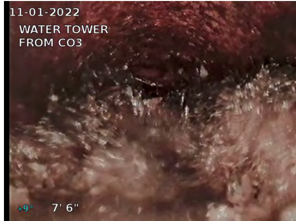
6, 00:01:01, 7.50ft Roots Medium Barrell from 3 o'clock to 9 o'clock, 50% of cross sectional area
