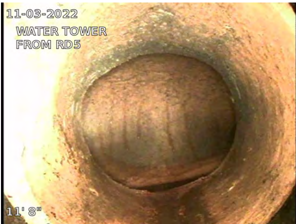
3, 00:00:26, 11.67ft Tee Connection / TIES INTO MAIN
