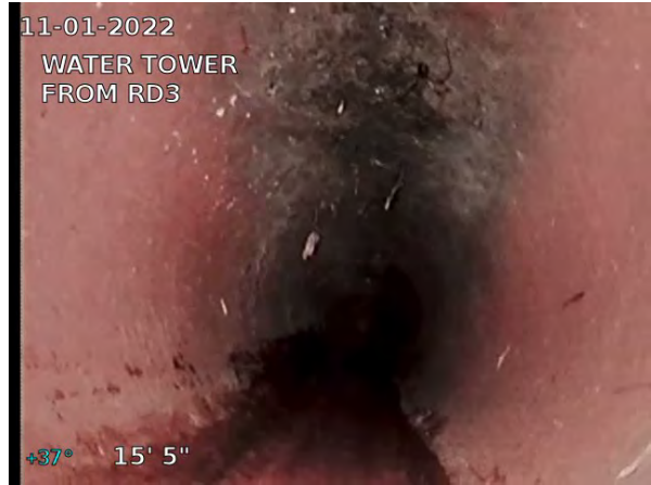
6, 00:00:49, 15.42ft Miscellaneous Shape or Size Change, dia/height: 6inch / TIED INTO 6 INCH MAIN
