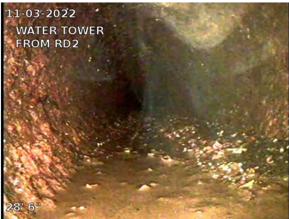
7, 00:01:09, 28.50ft Deposits Settled Fine, 5% of cross sectional area from 5 o'clock to 7 o'clock, within 8 inch, Start
