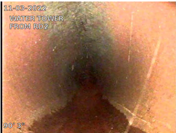
11, 00:02:57, 90.25ft Miscellaneous Material Change, Vitrified clay pipe / CHANGE TO VCP
