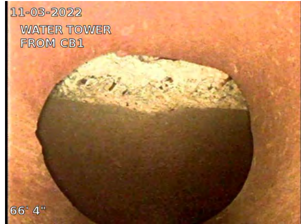
6, 00:02:01, 66.33ft Miscellaneous General Observation / TIES INTO 15 INCH MAIN
