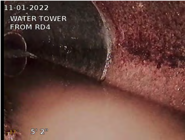
5, 00:00:25, 5.16ft Miscellaneous Shape or Size Change, dia/height: 6inch / TIES INTO 6 INCH MAIN
