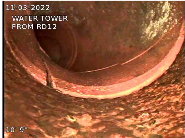
6, 00:00:34, 10.75ft Miscellaneous Material Change, Vitrified clay pipe / CHANGE TO VCP
