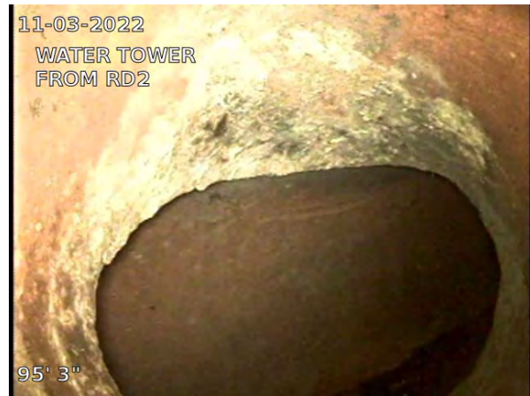
12, 00:03:09, 95.25ft Tee Connection / TIES INTO MAIN
