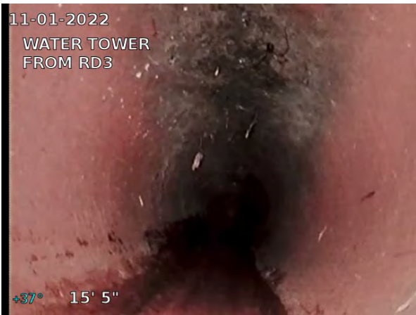
7, 00:00:49, 15.42ft Miscellaneous Material Change, Vitrified clay pipe / CHANGE TO VCP
