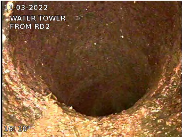
5, 00:00:48, 16.84ft Miscellaneous General Observation / LINE ANGLES DOWNWARD
