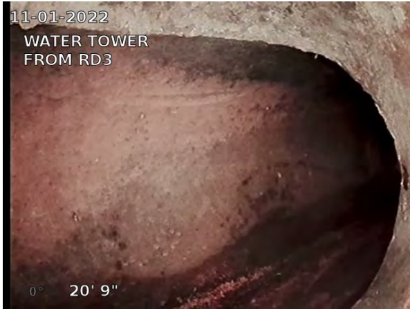
9, 00:01:09, 20.75ft Miscellaneous Shape or Size Change, dia/height: 8inch / TIES INTO 8 INCH MAIN
