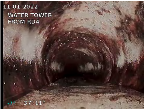
11, 00:01:51, 37.92ft Deposits Settled Fine, 10% of cross sectional area from 5 o'clock to 7 o'clock, within 8 inch, Start
