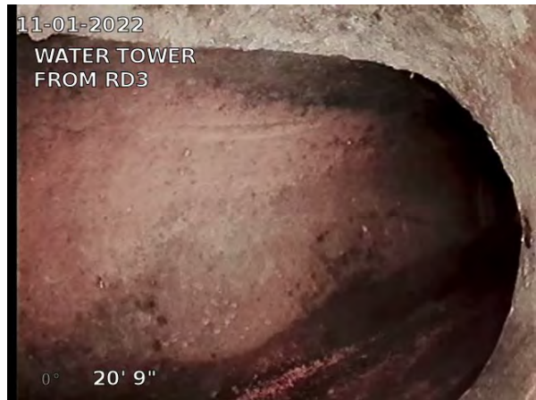
8, 00:01:09, 20.75ft Miscellaneous General Observation / WYE RIGHT INTO 8 INCH MAIN
