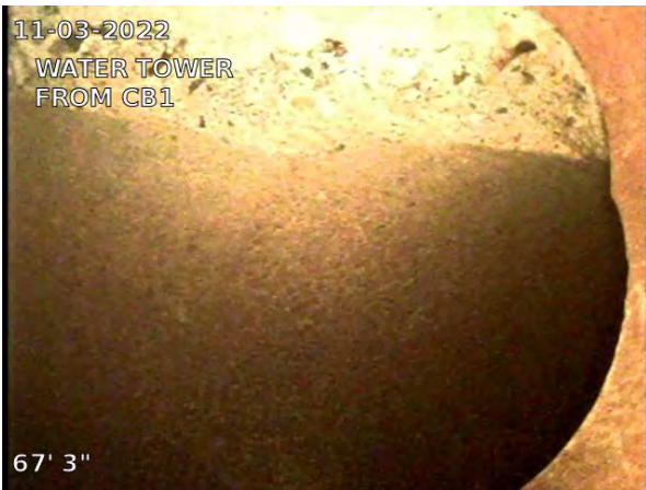
7, 00:02:03, 67.25ft Miscellaneous Shape or Size Change, dia/height: 15inch / TIES INTO 15 INCH MAIN
