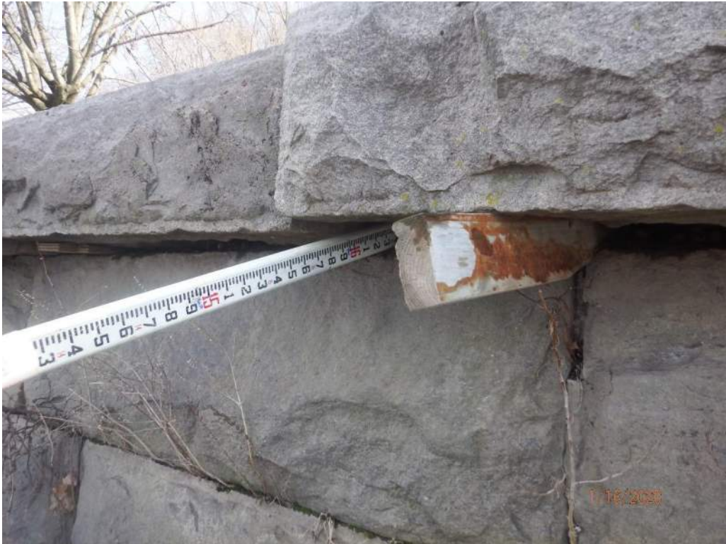
Photo 10: Timber shim installed between first and second course of stone
