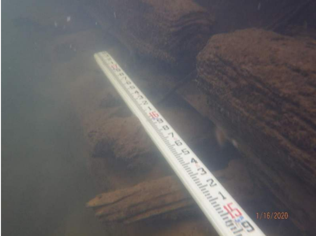
Photo 3: Typical view of the timber cribbing under the seawall.
