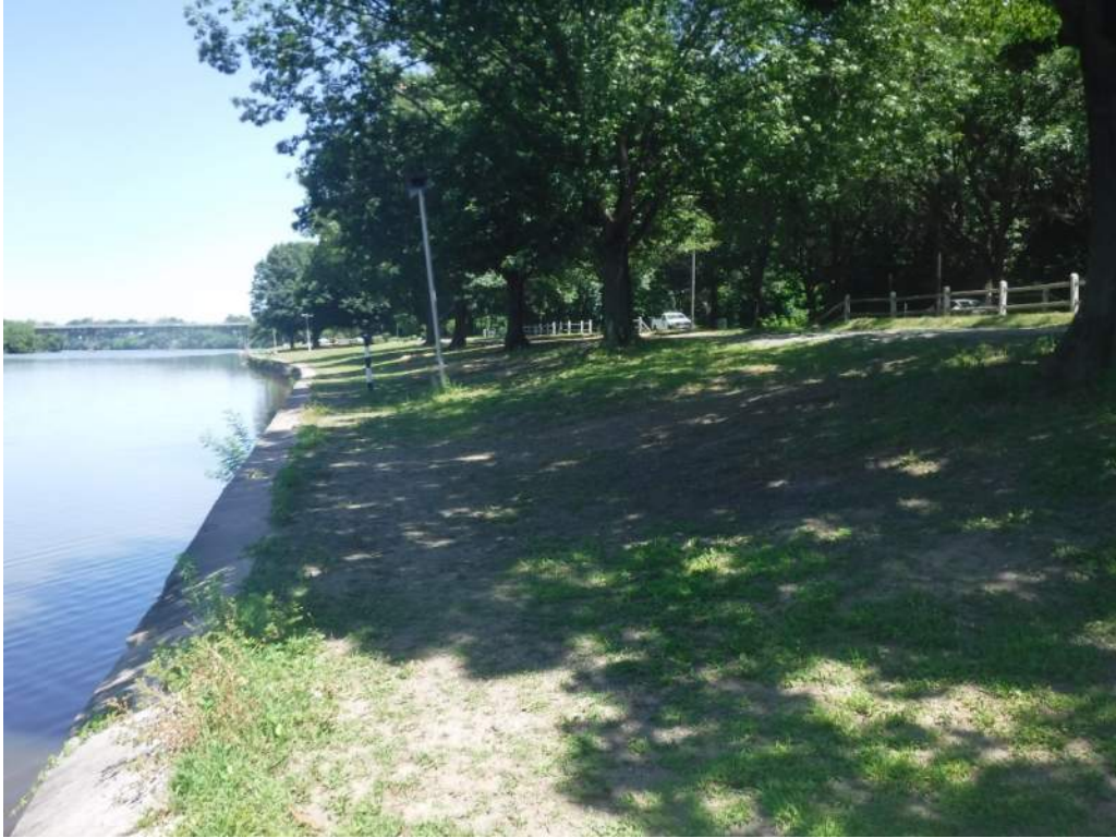
Photo 1: Marine wall view looking north towards Strawberry Mansion Bridge.
