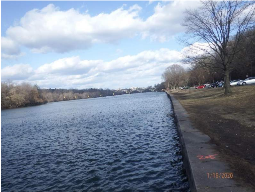
Photo 1: Seawall view looking north towards Strawberry Mansion Bridge.
