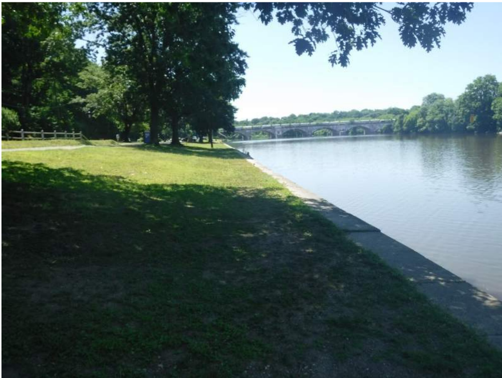
Photo 2: Marine wall view looking south towards reviewing stands.
