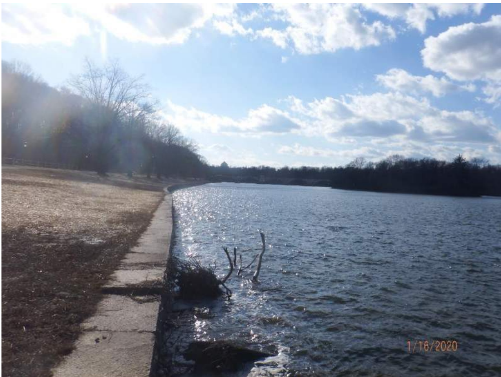
Photo 2: Seawall view looking south towards reviewing stands.
