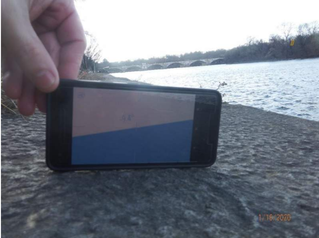
Photo 9: Top row of blocks settled up to 9.4 degrees towards the river
