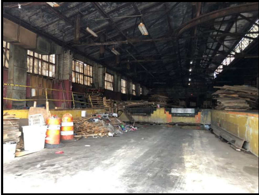
Photograph 5 – Inside building east of the property
