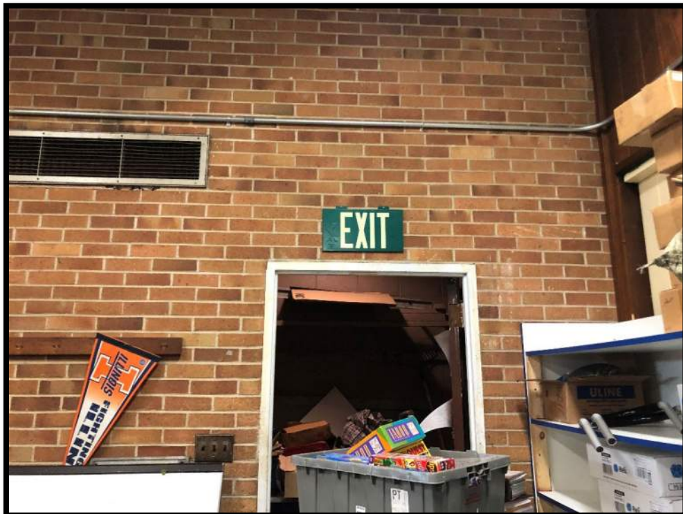
Photograph 10 – Main room area, used as storage, and entry to storage room
