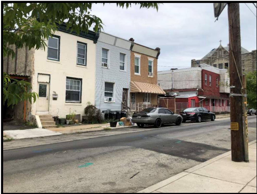
Photograph 6 – Facing south, showing residential, retail and church buildings
