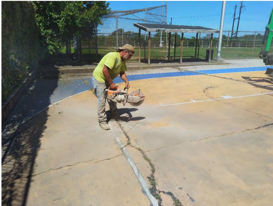
Photo 8: Third test pit on high side of wall
