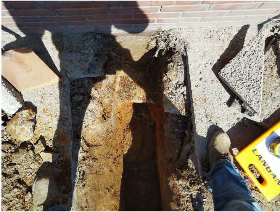
Photo 4: Top view of test pit on low side of wall
