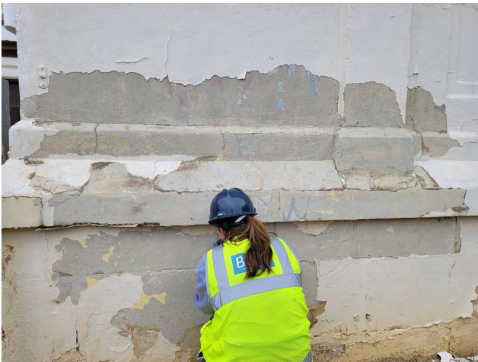
Figure 9. Paint removal test location after mechanical paint removal. Approximately three to four layers of overpaint remained on most of the surface.
