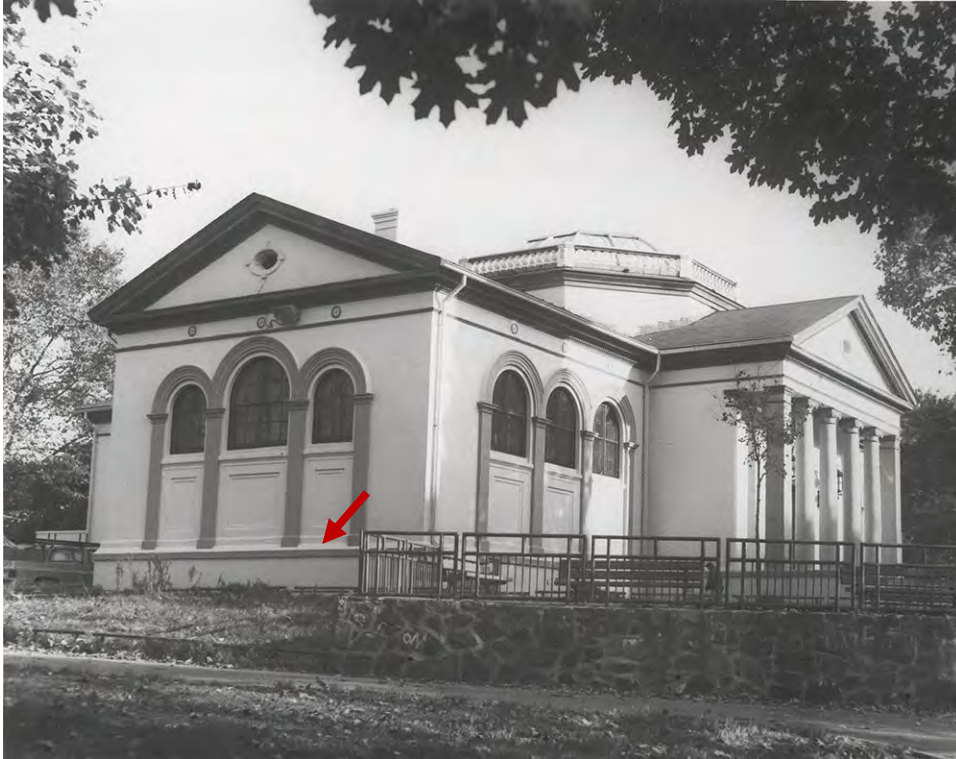
Figure 7. Image of the renovated library in 1975. This is the earliest image that captures the stucco slope installed above the belt course (arrow). Compare to Figure 6, where the top of the projecting belt course is flat. Image Credit: Free Library of Philadelphia Digital Collections.
