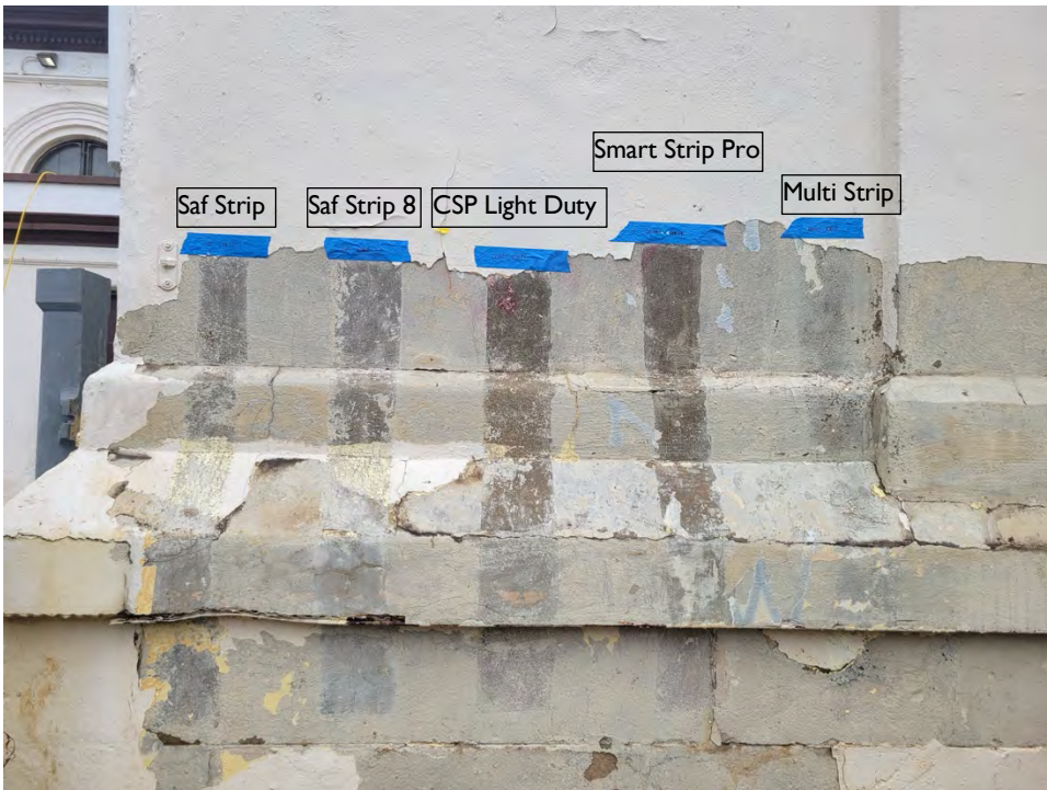
Figure 11. Paint removal test at completion. The CSP Light Duty and Smart Strip Pro performed the best, removing most of the remaining paint layers to reveal the brownish gray stucco skim coat.
