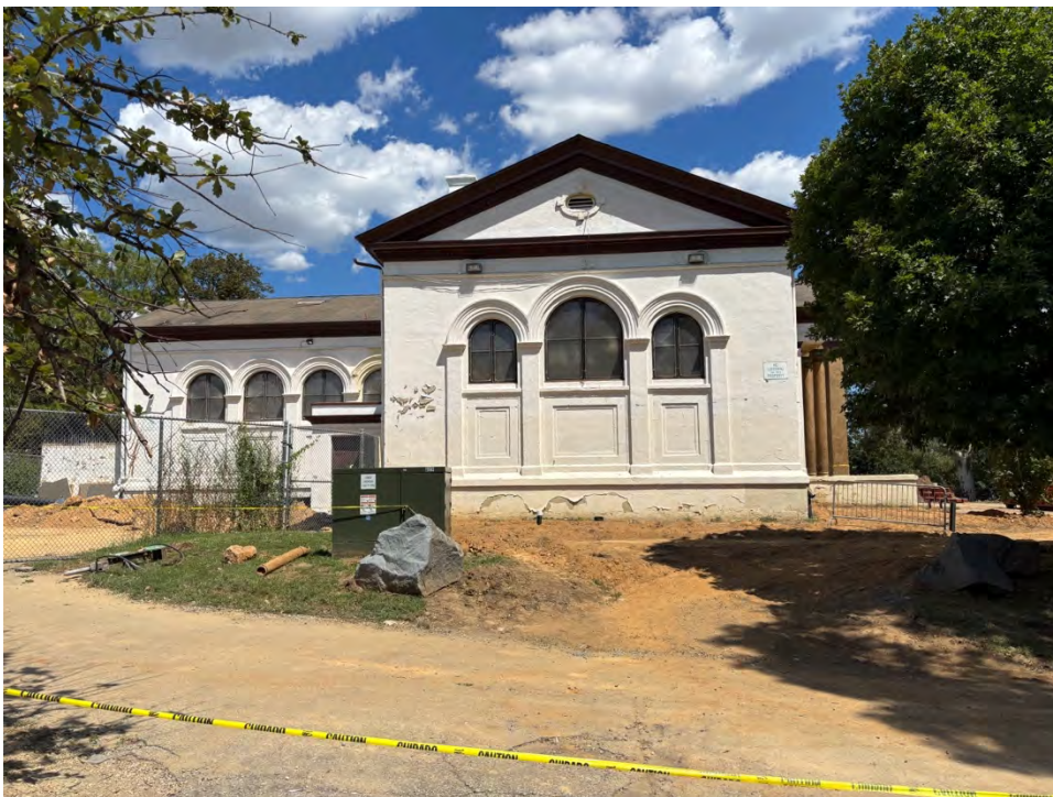
Figure 4. McPherson Square Library, southwest elevation.
