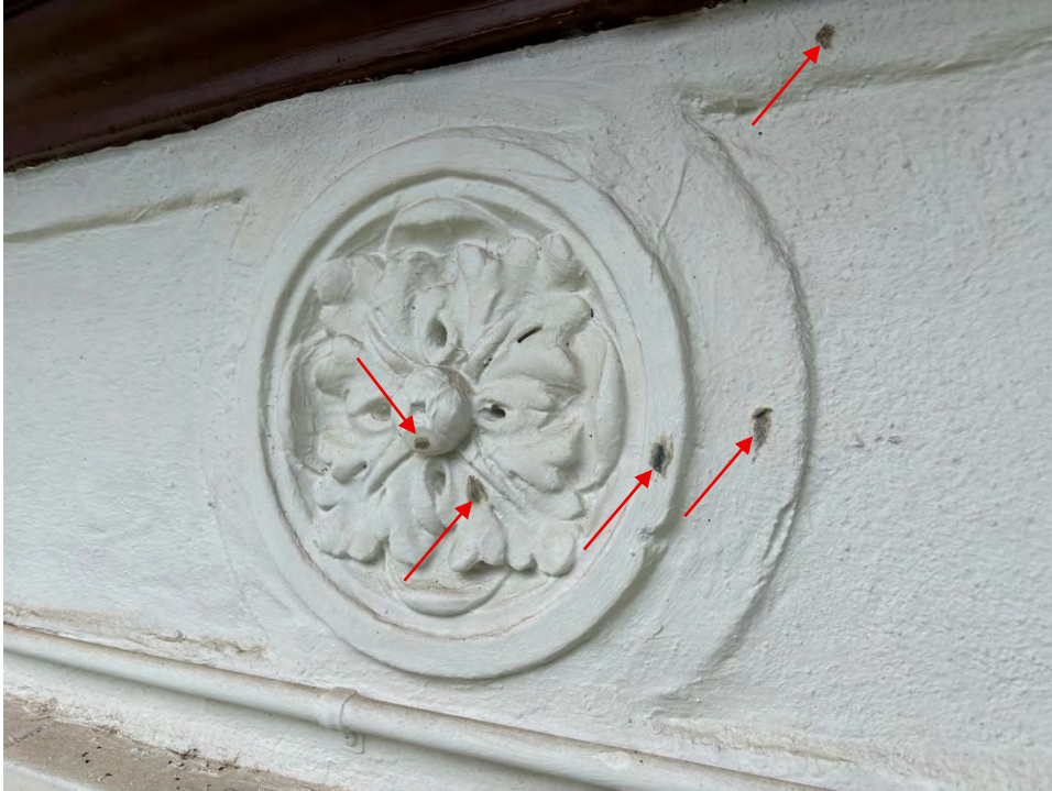
Figure 24. Field investigation was performed on the terra cotta rosette and surrounding moldings by scraping away to overpaint to observe the substrate and number of paint layers present. All terra cotta elements appear to have a dark brown or dark green glaze (arrows).
