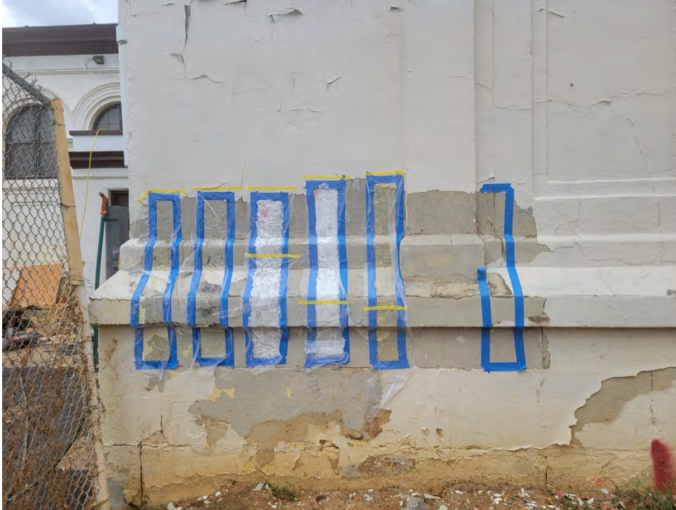
Figure 10. Five chemical paint removers were tested on the left side of the pilaster. Each test location measured approximately 10" x 3.5'.
