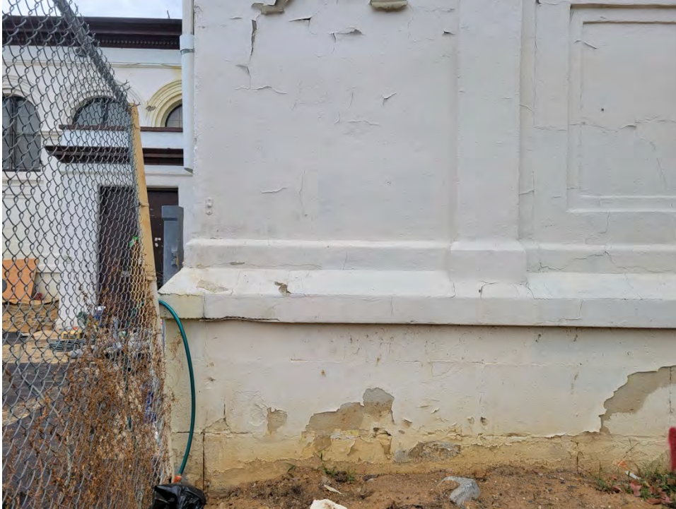
Figure 8. Paint removal test location on the southwest elevation, before testing.
