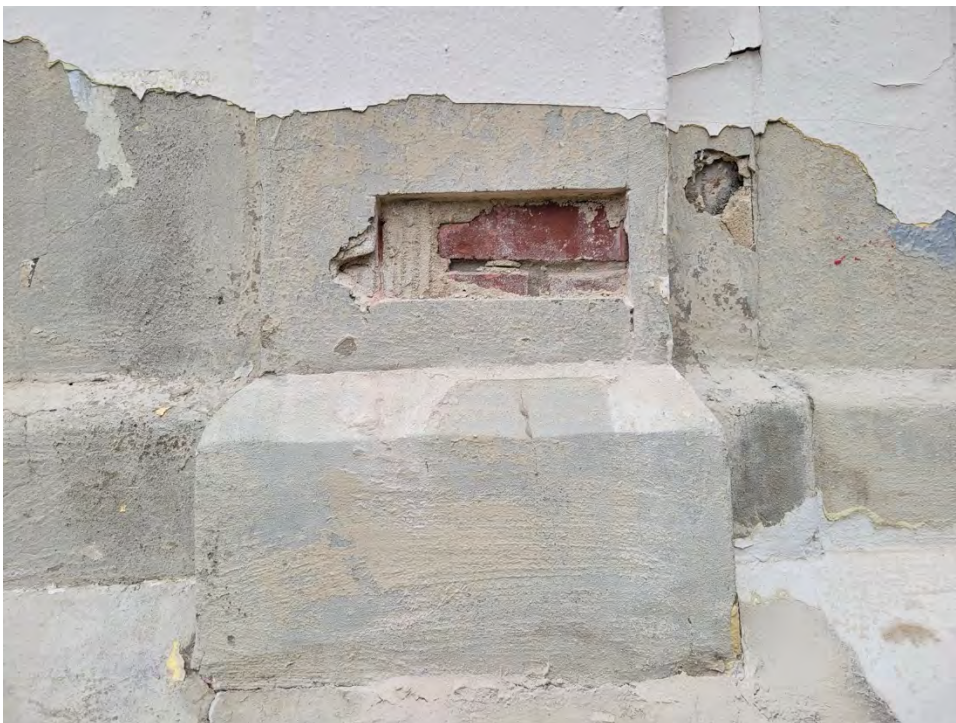
Figure 28. The stucco sample was removed from a pilaster on the southwest elevation.
