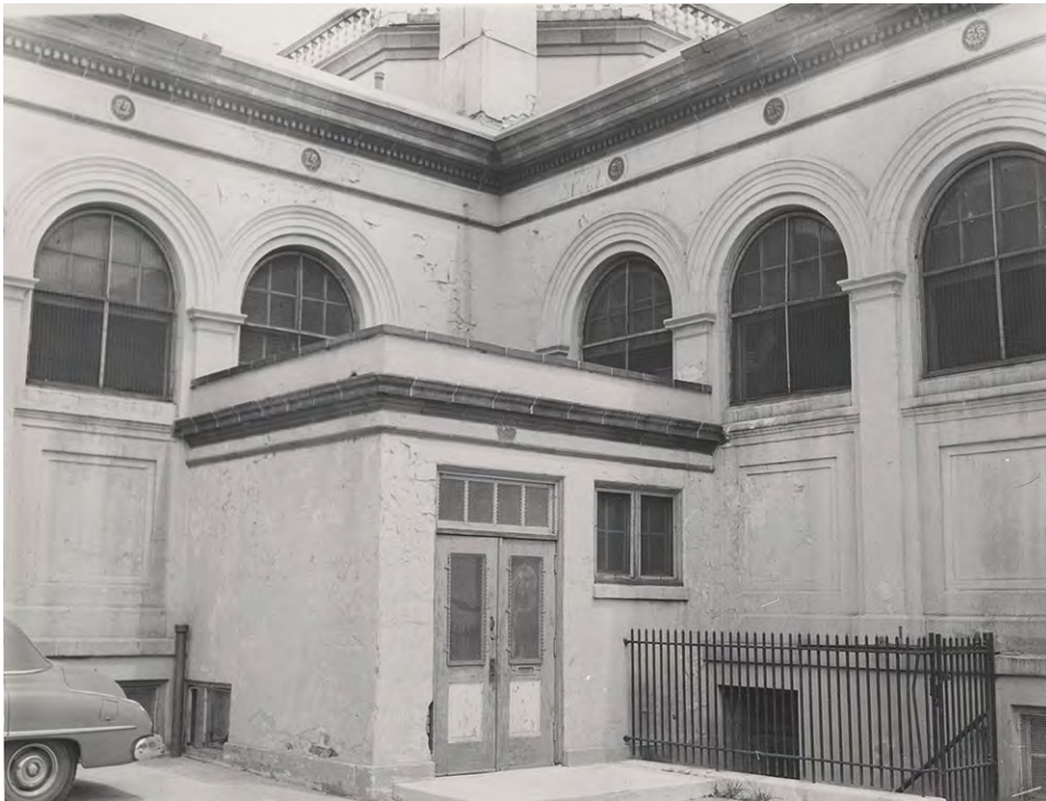
Figure 6. Rear entrance to the library at the northwest elevation, view looking east, late 1950s. Note the flaking paint on the walls. This is the earliest image in which the building is clearly painted. Image Credit: Free Library of Philadelphia Digital Collections.
