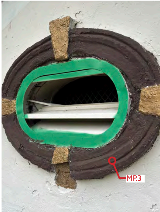
Figure 2. Louvered oval window
