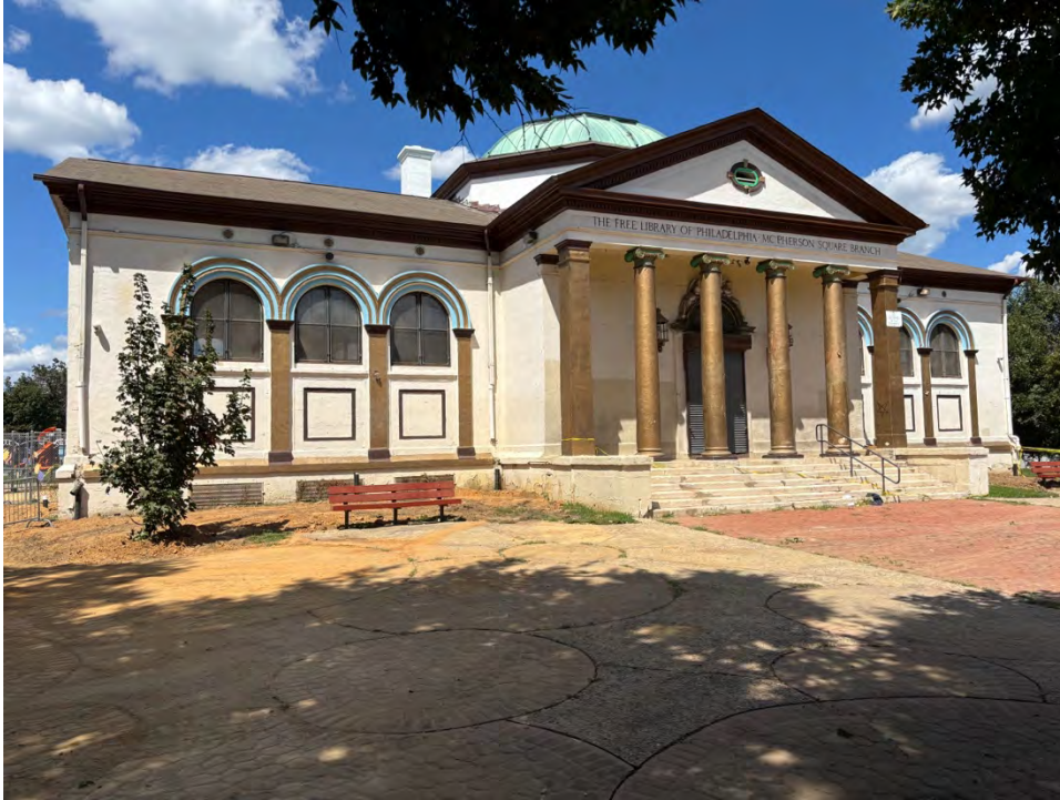
Figure 1. McPherson Square Library façade (southeast elevation).
