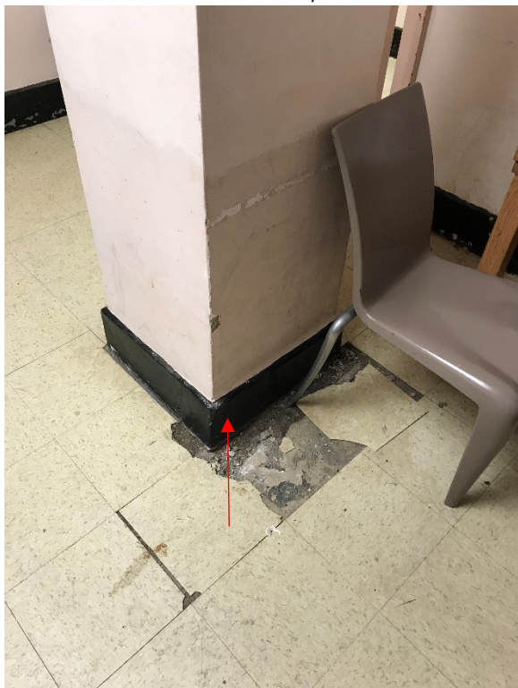
Cement Cove Base in the Basement verified non-asbestos
