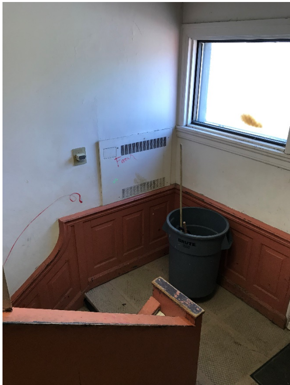
Rear Entrance Foyer – No ACM identified behind recessed radiator
