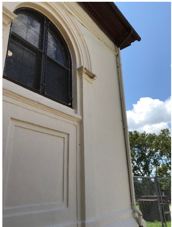
Coating applied to Exterior Stucco verified non-asbestos
