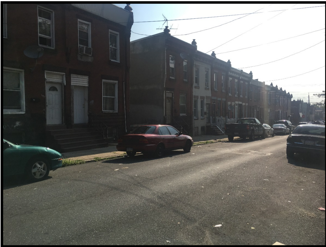
Photograph 2: Northern Adjoining Sites: Residential Row Houses.
