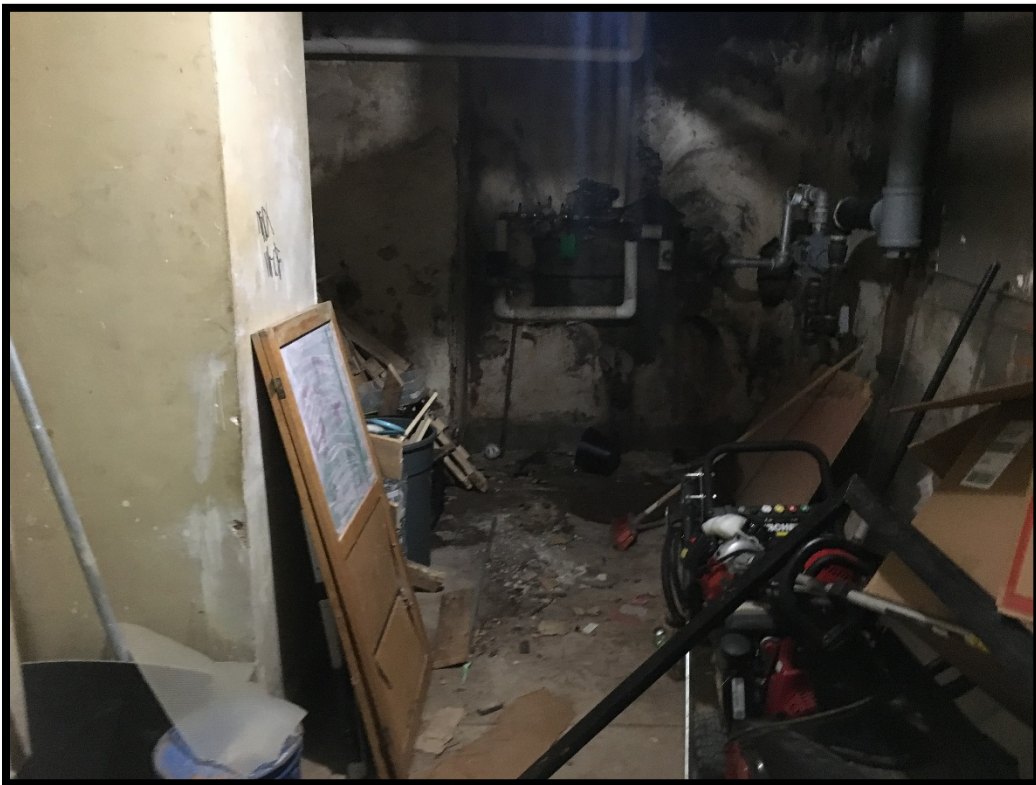
Photograph 10: Storage room in the Basement.
