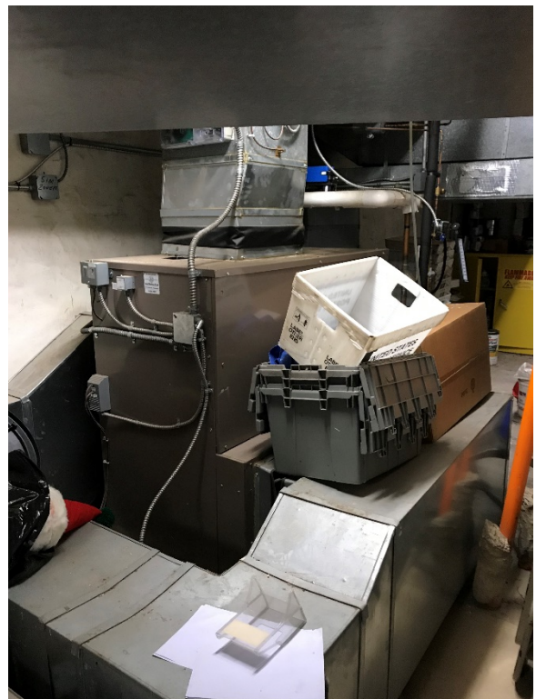
No asbestos identified with Air Handling Units 1 and 2. Black Vinyl Vibration Damper Connectors present
