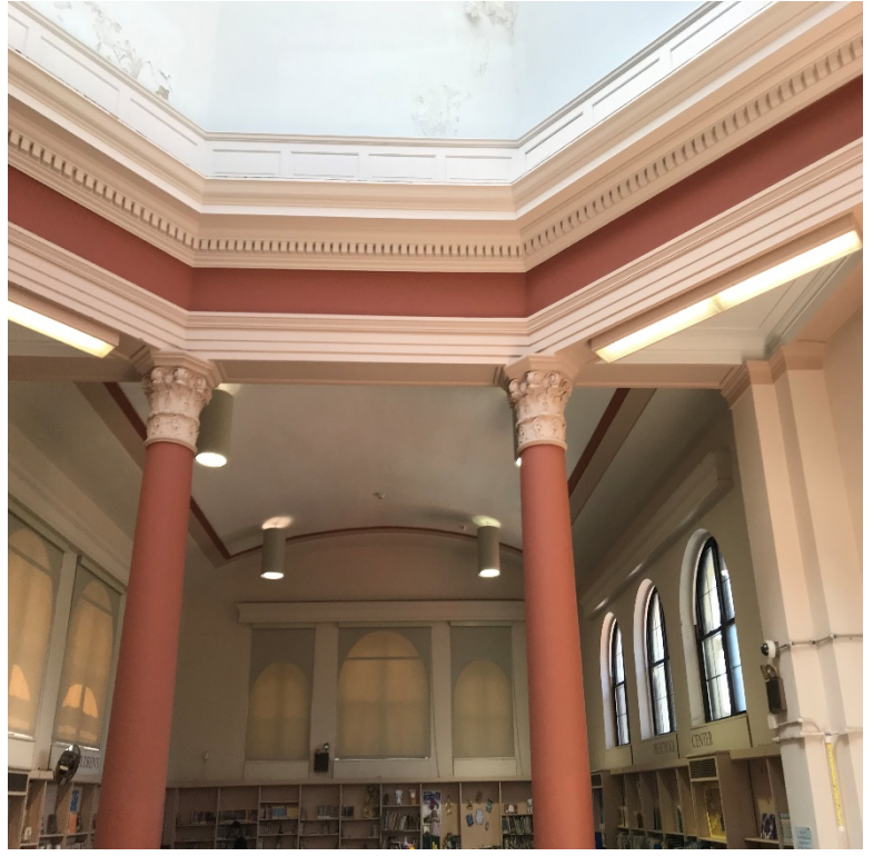
All Plaster Walls, Ceilings and Columns verified non-asbestos throughout the Building
