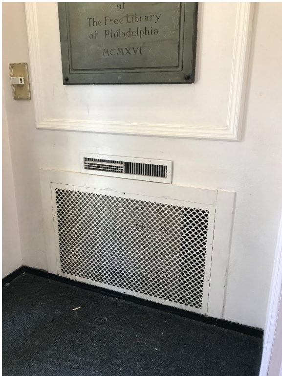
First Floor Entrance Foyer – No ACM identified behind recessed radiator
