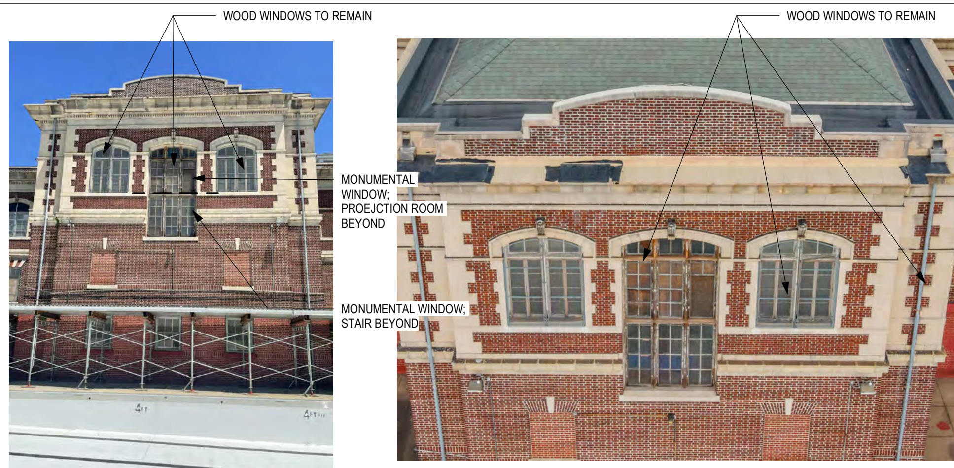
WOOD WINDOWS TO REMAIN - EXTERIOR
