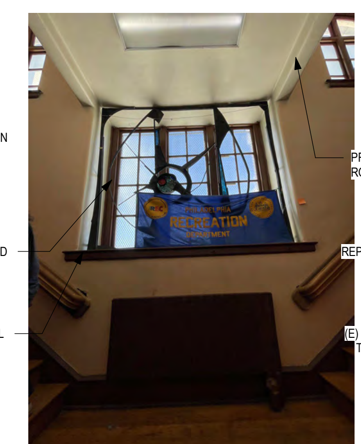
MONUMENTAL WOOD WINDOW - INTERIOR - LOWER HALF AT STAIR
