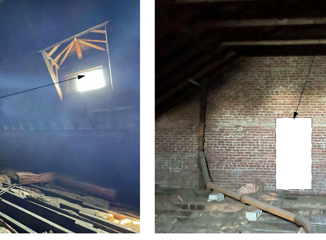
ATTIC - SOUTH WING - NORTH WALL
