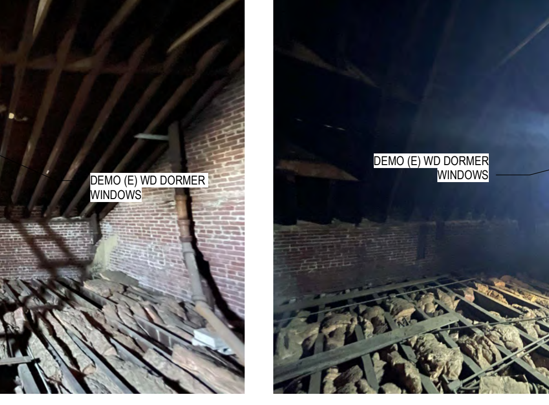
ATTIC - SOUTH WING - SOUTH WALL
