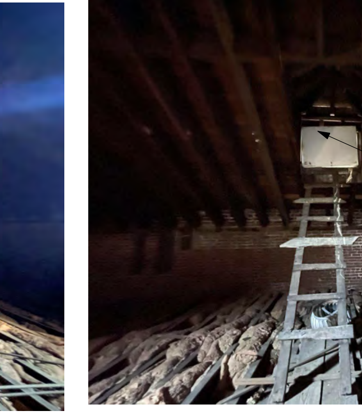
ATTIC - SOUTH WING - WEST WALL
