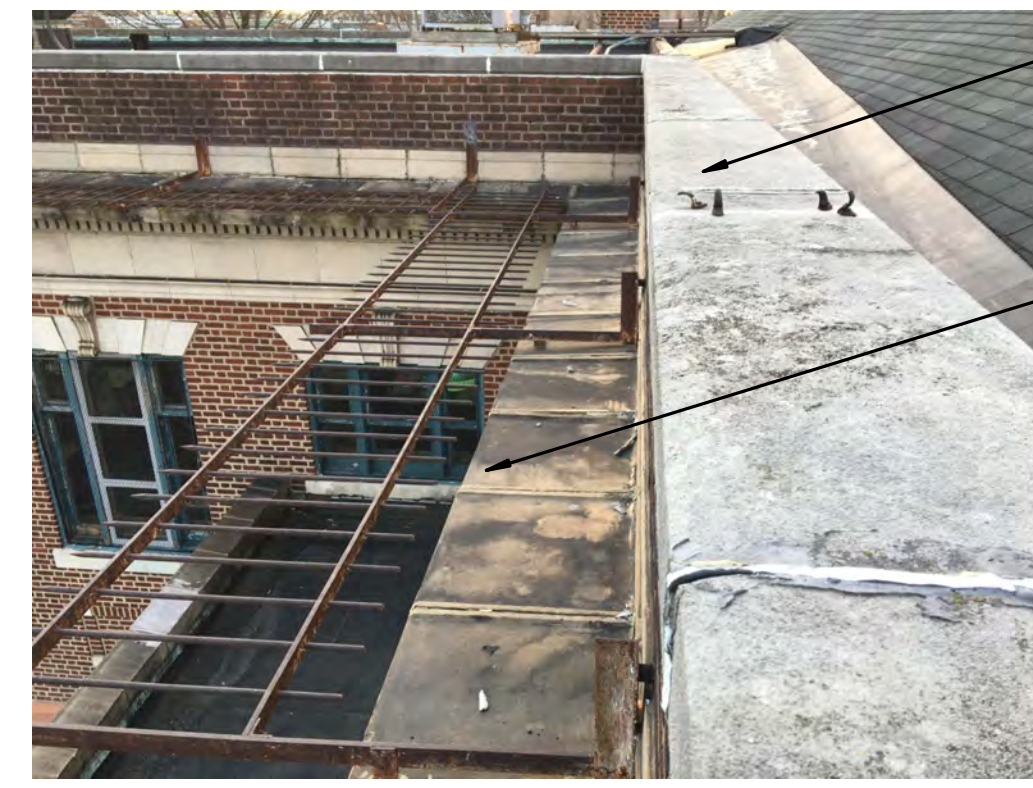
7 ROOF CONDITION - GRILLE
