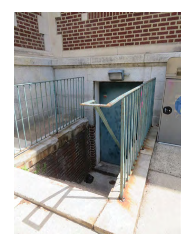
④ AD-15 LOWER STAIR
