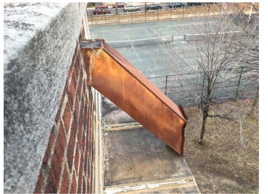
6 ROOF CONDITION - SCUPPER
