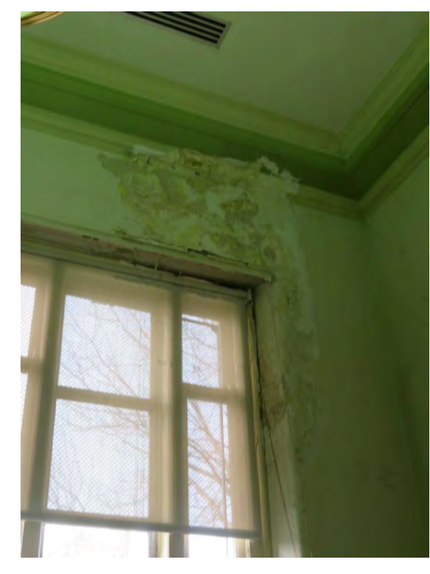
11 INT PLASTER REPAIR
