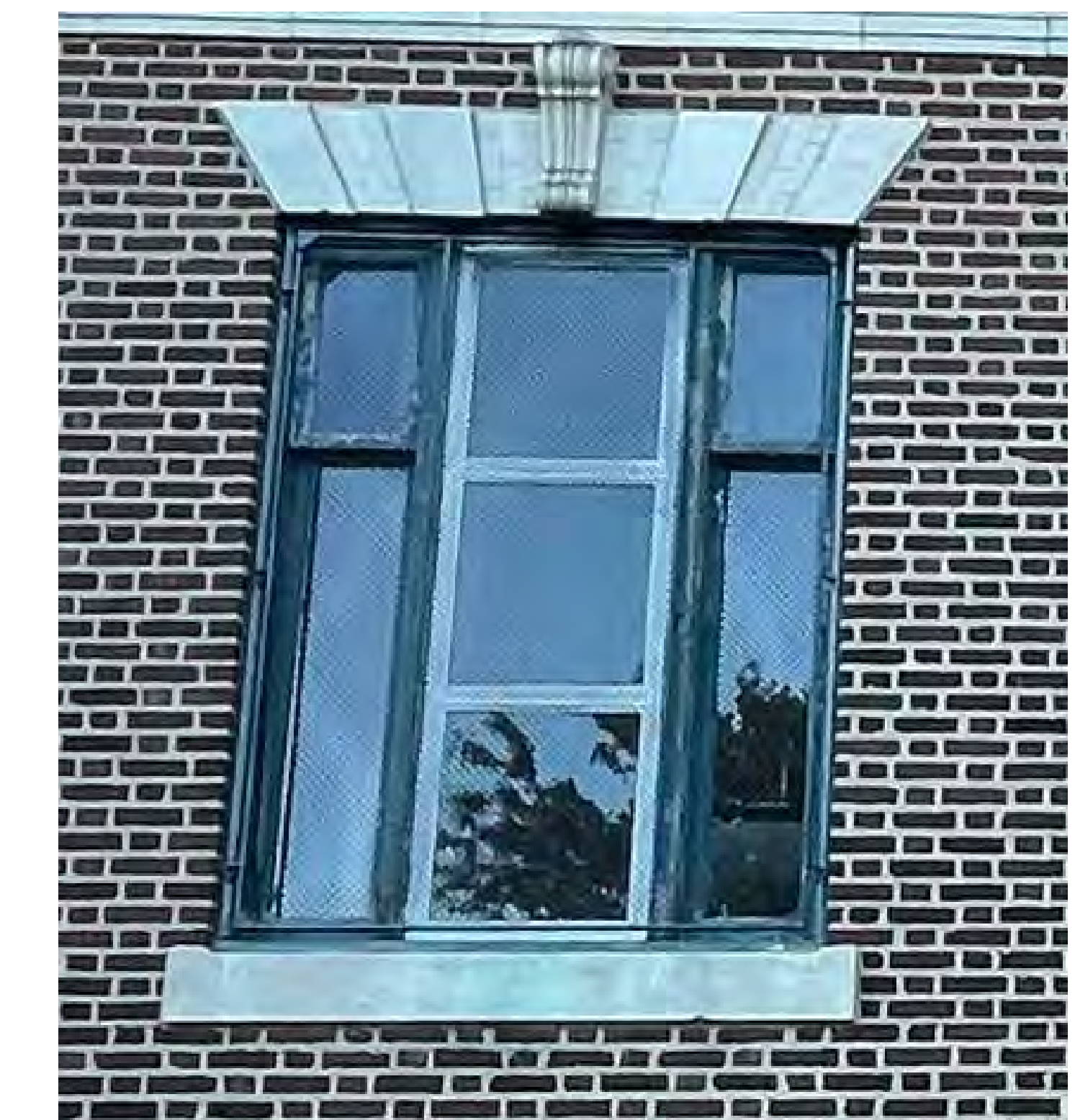
7 EAST ELEV. WINDOW CONDITION TYP ALL 1ST FLOOR WINDOWS SEE SCOPE OF WORK WM AND WS
