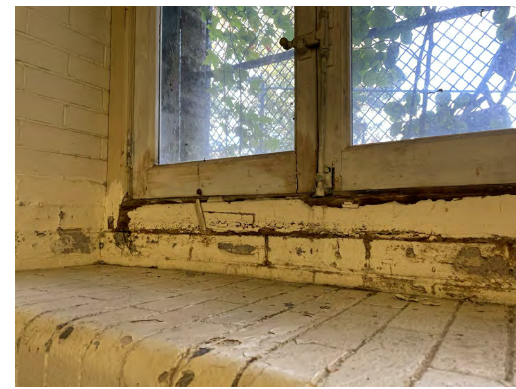
4 WINDOW SILL - MEETING ROOM - LOWER LEVEL
