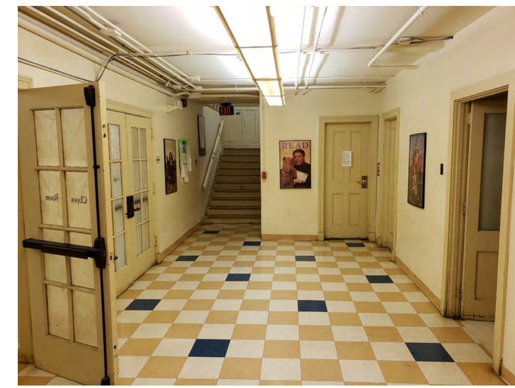
2 CORRIDOR - LOWER LEVEL
