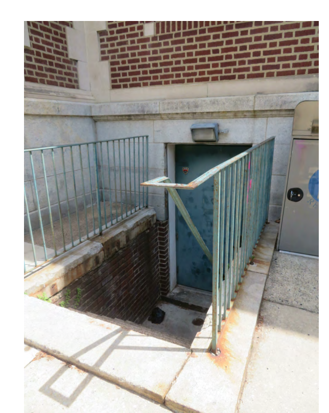
4 AD-15 LOWER STAIR
