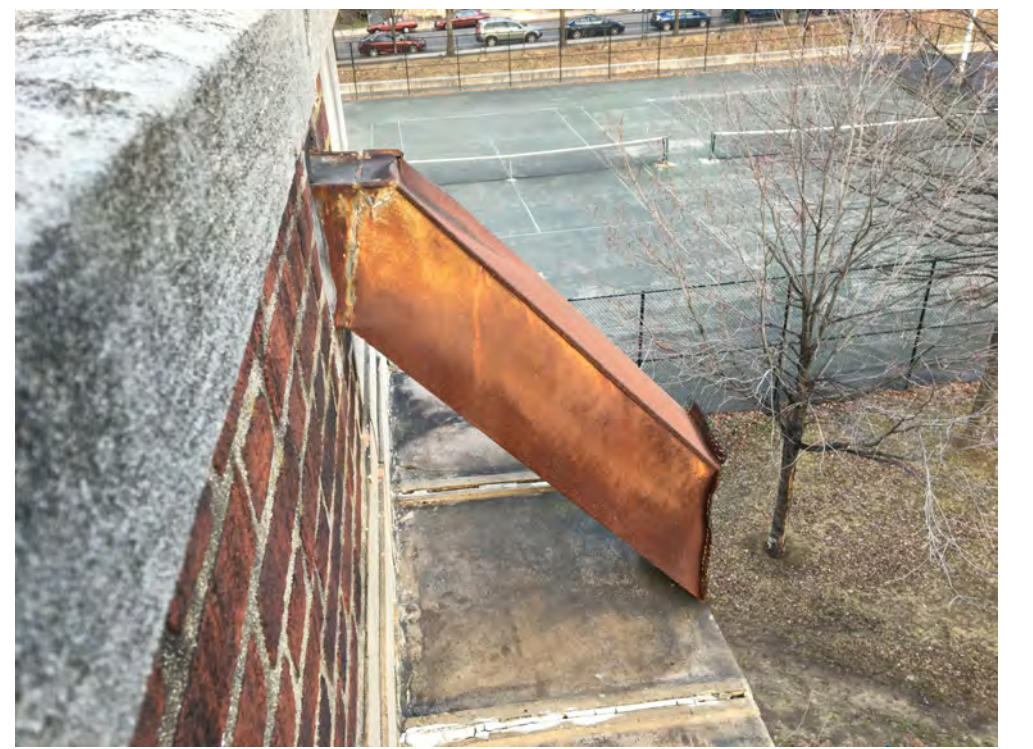
6 ROOF CONDITION - SCUPPER
