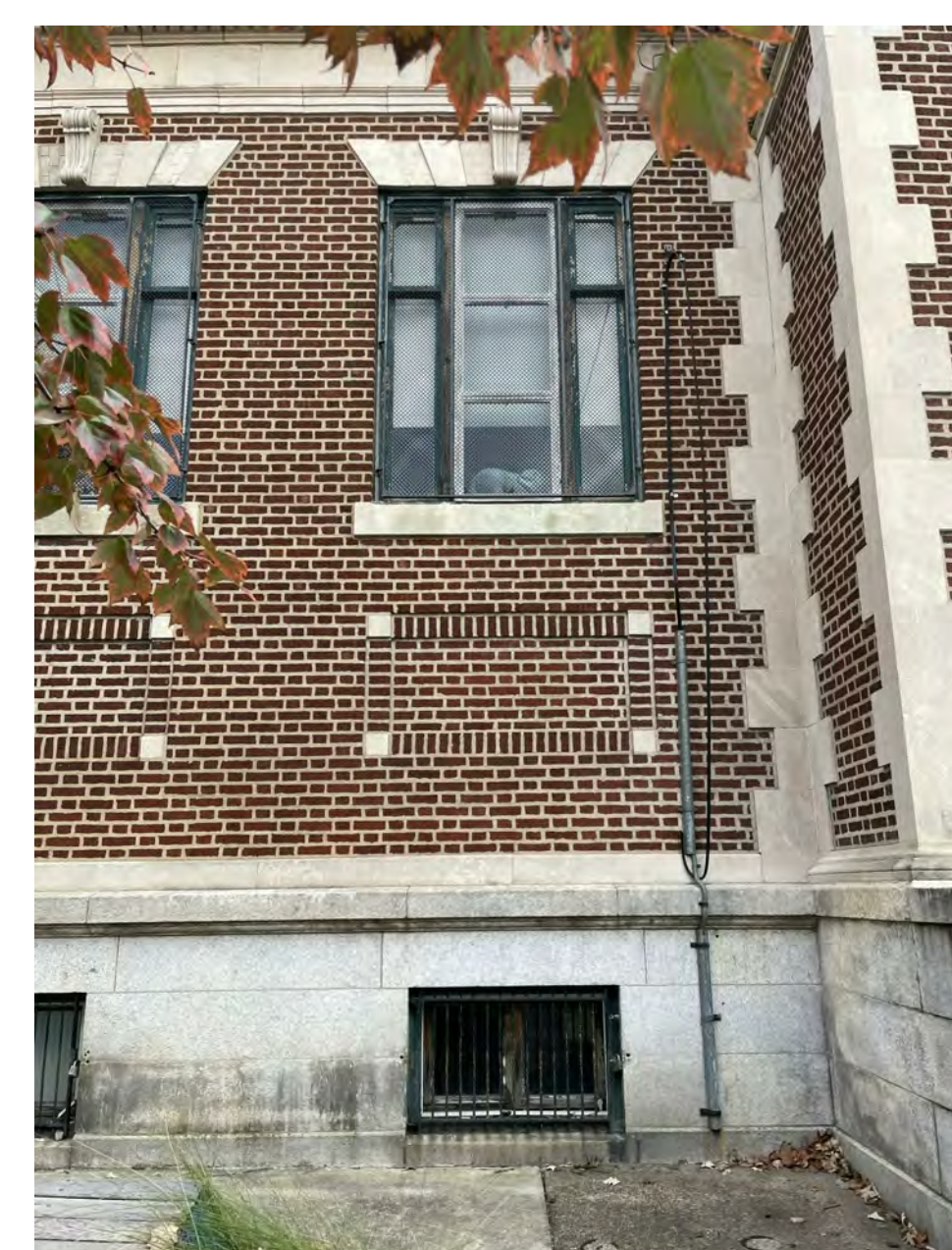
3 WEST ELEV - CONDUIT TO BE REMOVED 12" = 1'-0"
