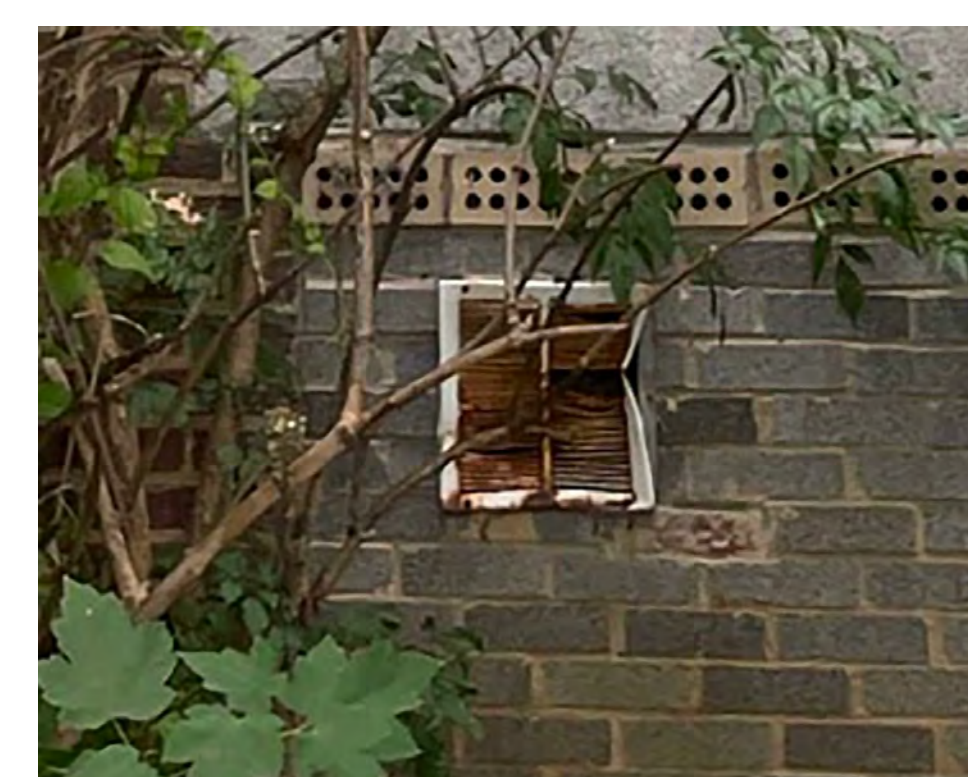
10 L.L FACADE CONDITION - SOUTH - WDW 010
