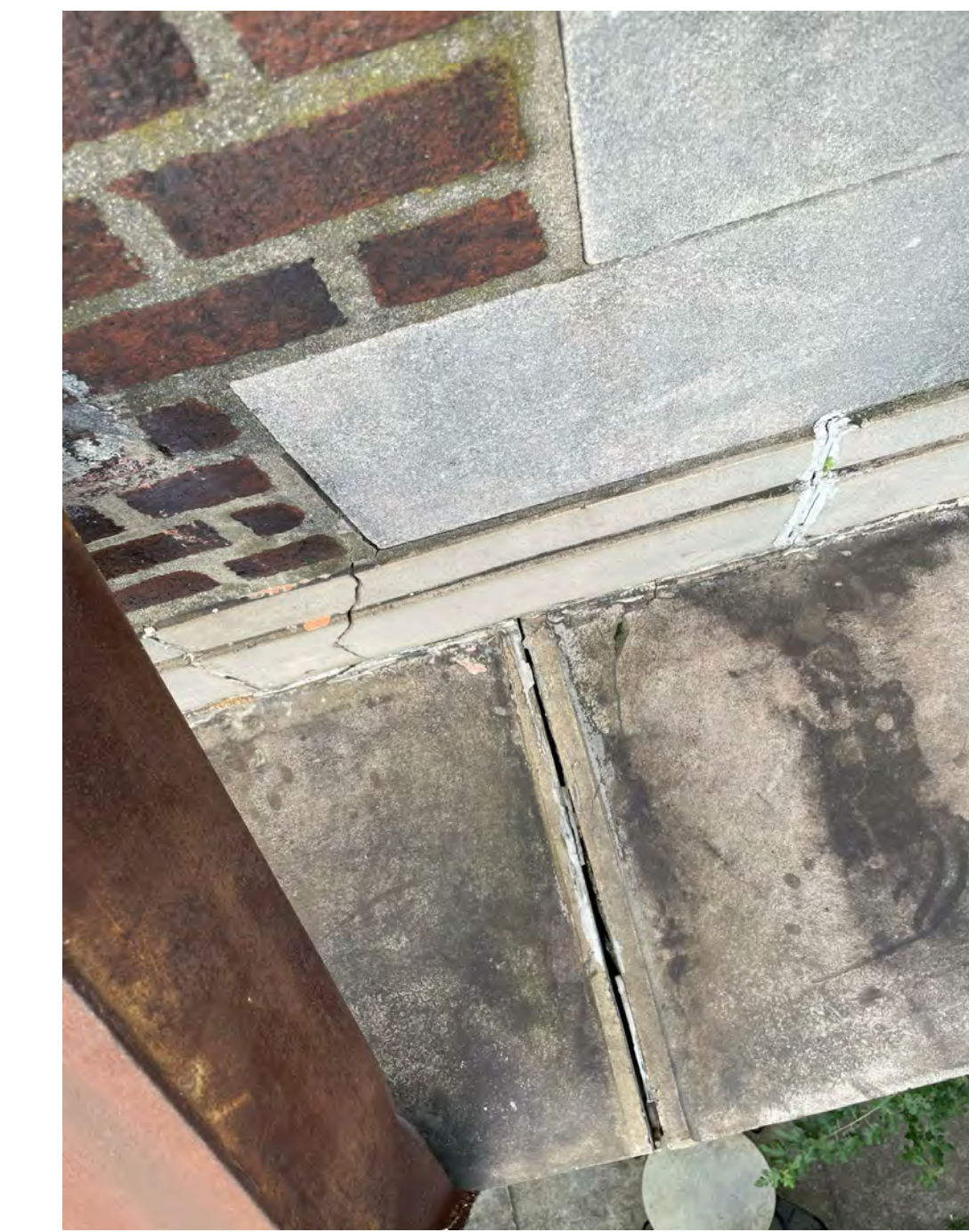
8 ROOF CONDITION - TERRACOTTA CORNICE
