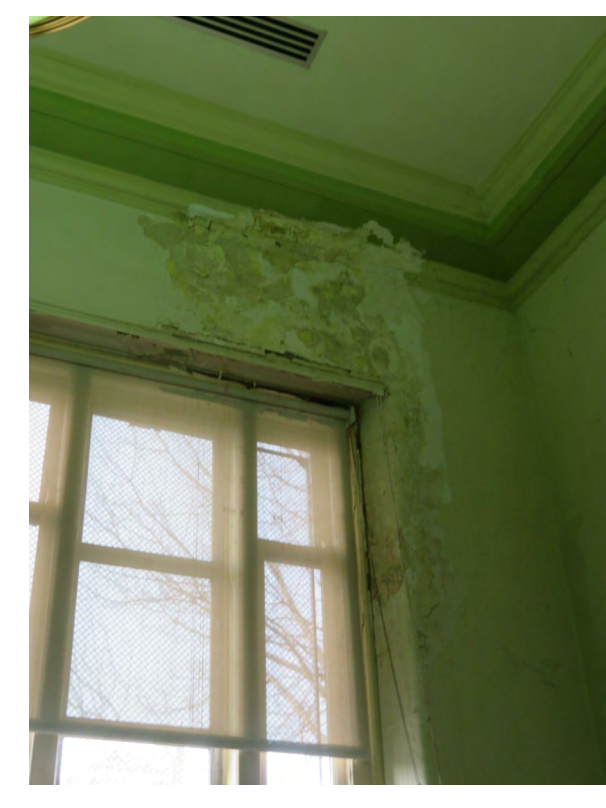
11 INT PLASTER REPAIR
