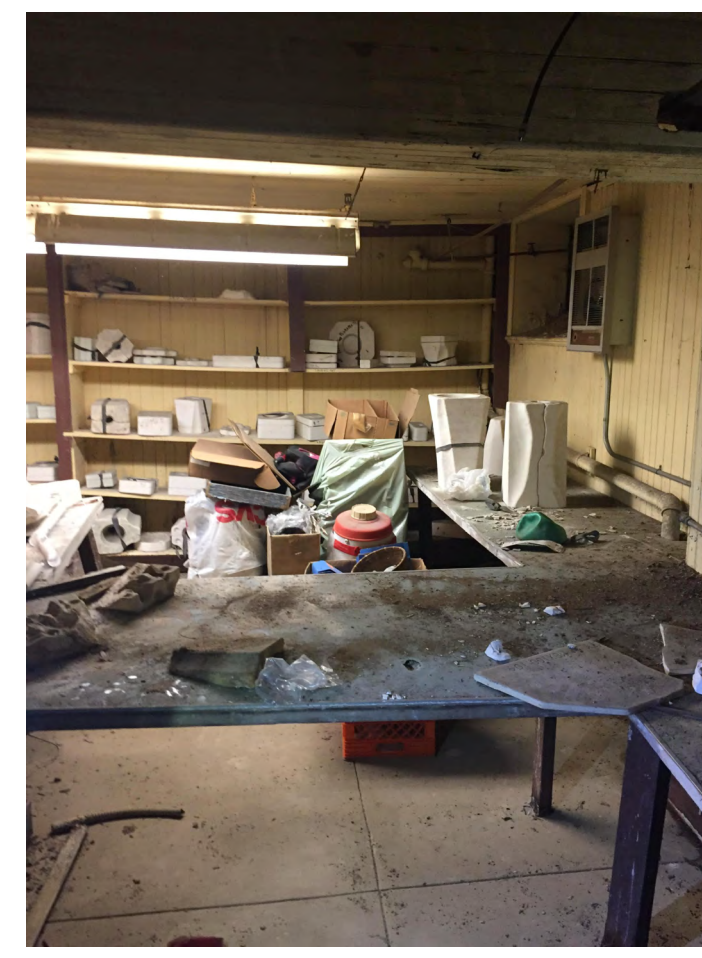
EXISTING REC BUILDING BASEMENT (CERAMICS ROOM)
