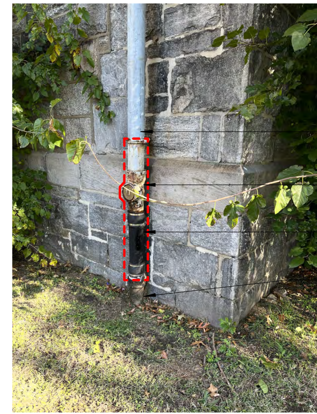
EXISTING DOWNSPOUT REPAIR/REPLACEMENT
