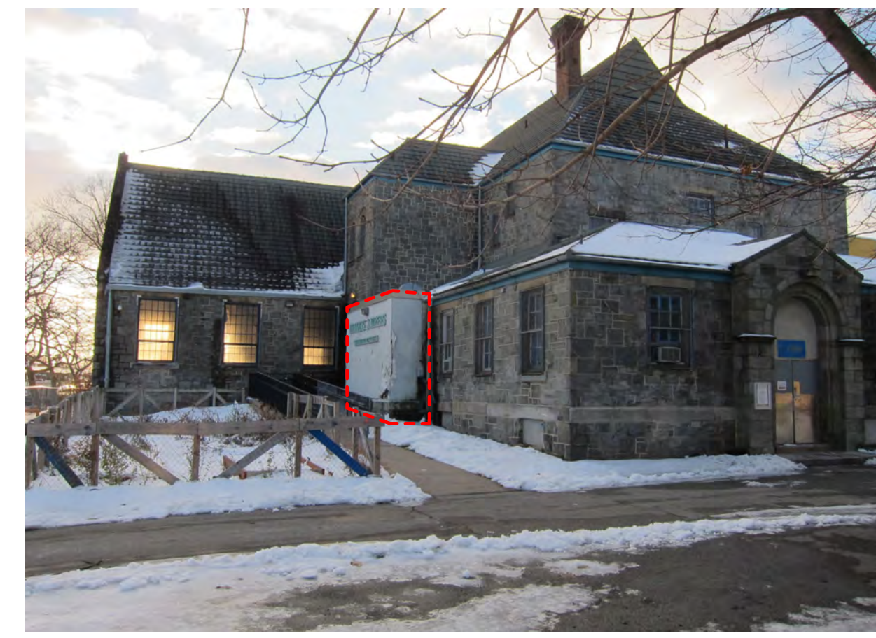
EXISTING BATHROOM ADDITION TO BE DEMOLISHED
