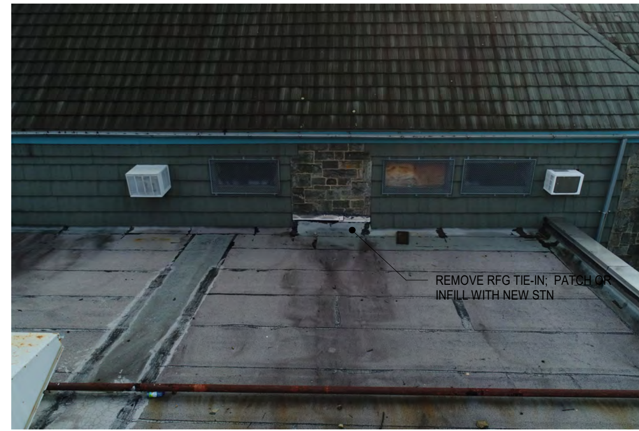
EXISTING REC BUILDING NORTH ELEVATION CLADDING TO BE SELECTIVELY DEMOLISHED ABOVE GYMNASIUM
