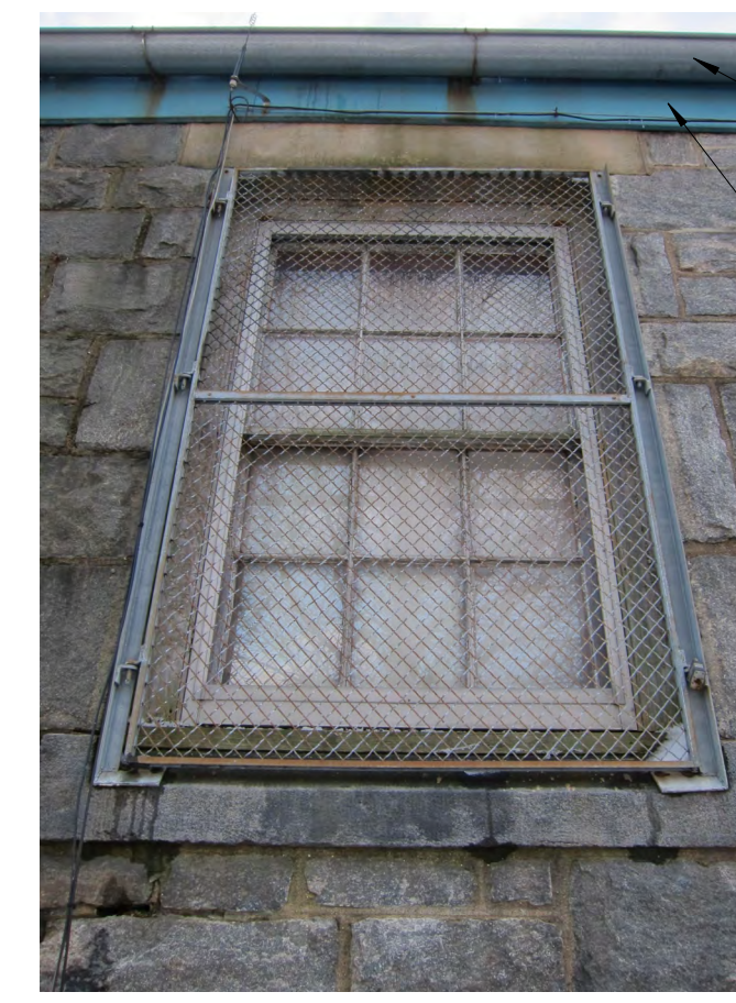
(E) HALF ROUND GUTTER, REFER TO DEMO ELEVATIONS FOR EXTENT OF REPLACEMENT (E) FASCIA BD TO BE CLEANED & PAINTED, TYP.
