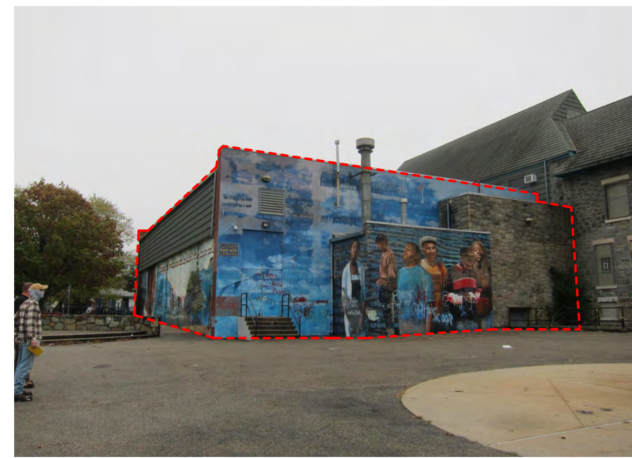
EXISTING GYMNASIUM BUILDING ADDITION TO BE DEMOLISHED, LOOKING EAST
