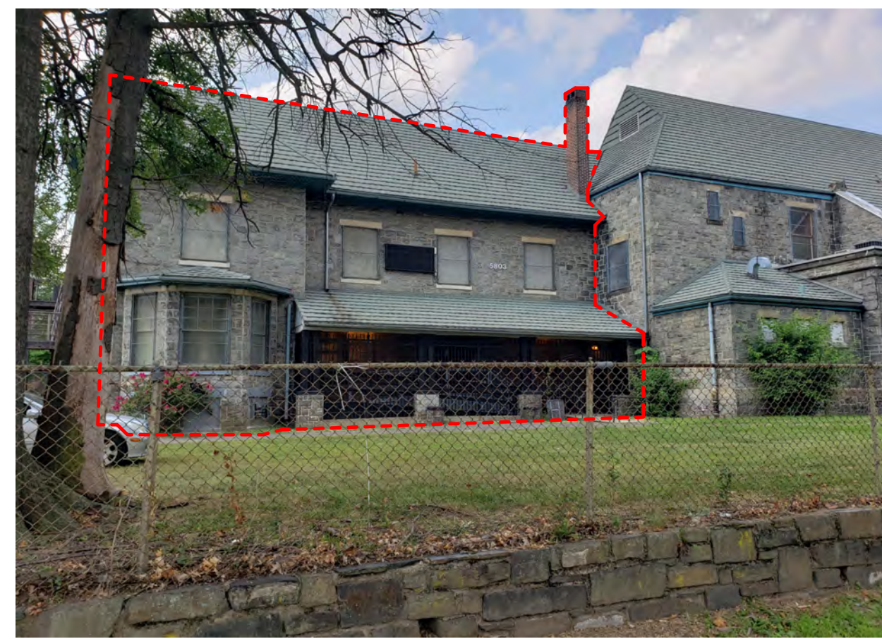
EXISTING ANNEX BUILDING ADDITION TO BE DEMOLISHED, LOOKING NORTH
