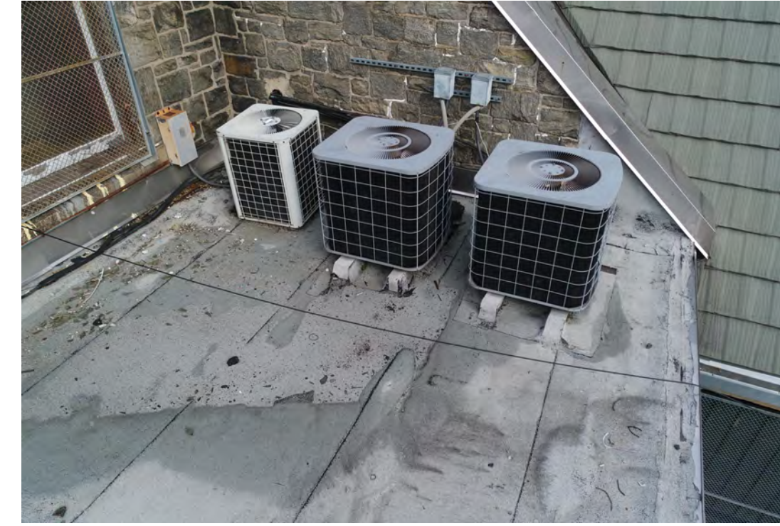
EXISTING ROOFTOP EQUIPMENT TO BE DEMOLISHED
