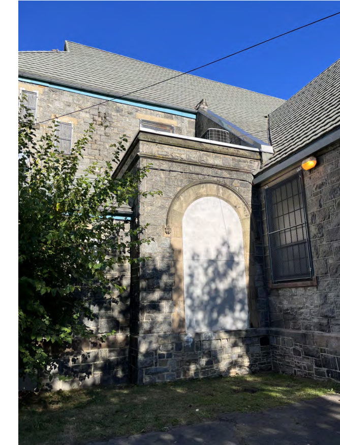
VIEW LOOKING NORTH @ EXG INFILL
