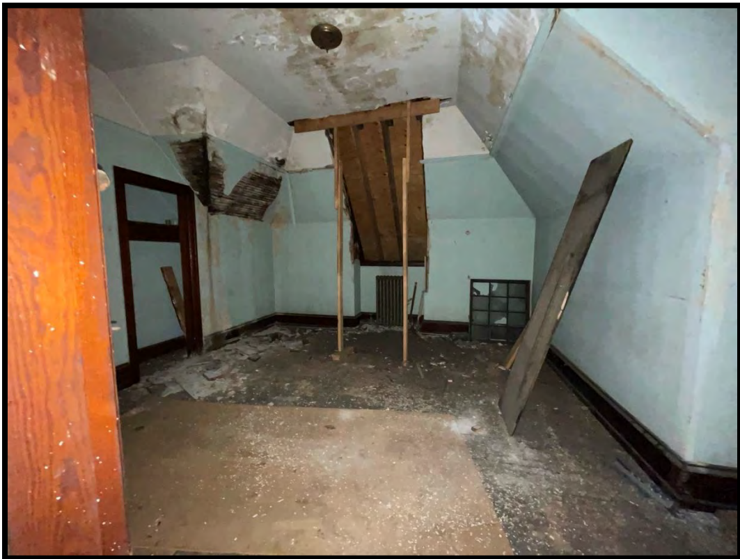
Photograph 26: Third floor of Annex.
