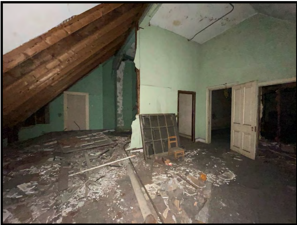
Photograph 20: Third floor of the building.
