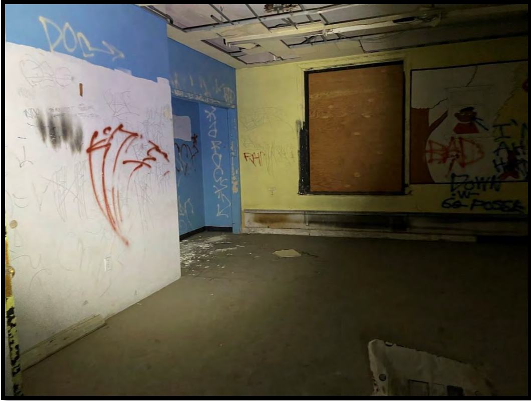
Photograph 25: Second floor of Annex.
