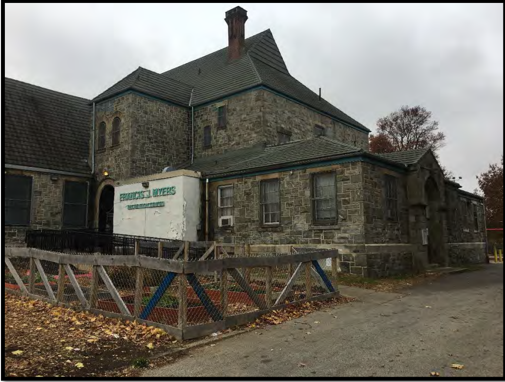
Photograph 1: View of Recreation Center facing southwest.
