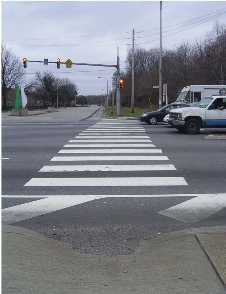
Existing Crossing of 84th Street
