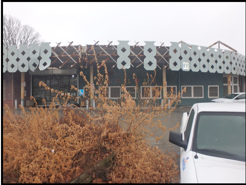
Photograph 1 – Carousel House Front Entrance, from Avenue of the Republic, facing south.
