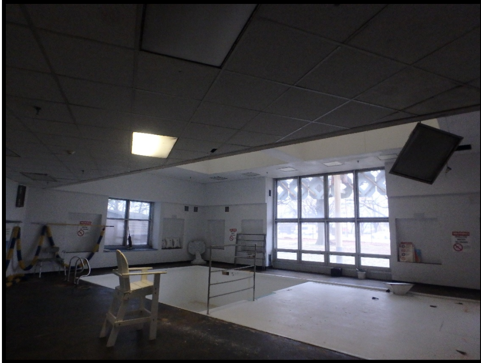
Photograph 11 – Pool area with an office, utility rooms, chemical storage and bathrooms.
