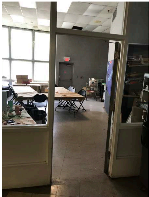
Insulation inside Wood and Metal Fire Doors throughout (assumed present; assumed asbestos-containing)
