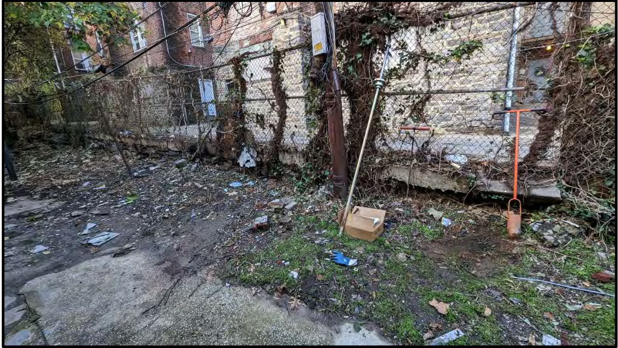
Photo 13: GF-7 looking northwest showing decreasing height of retaining wall
