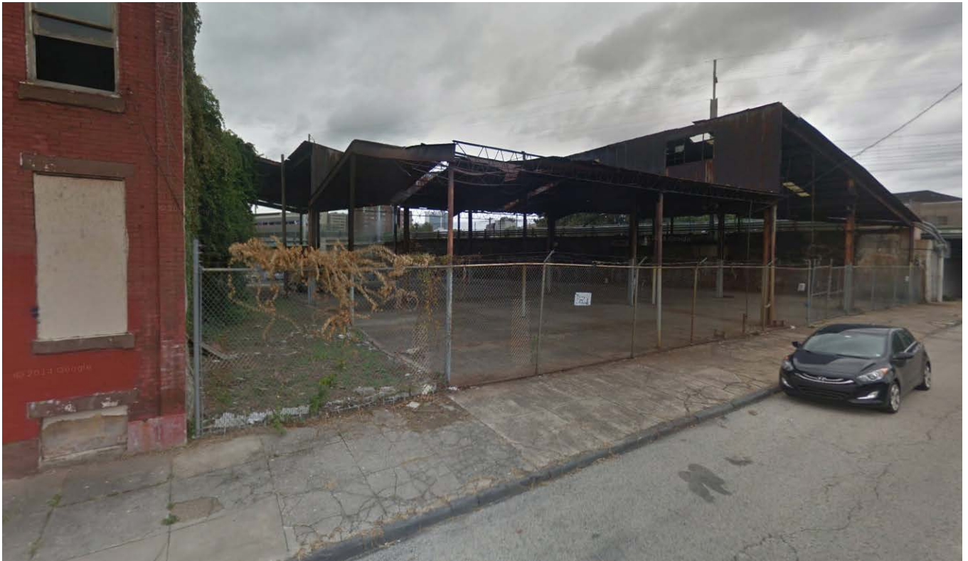
1018-1030 W. Colona Street (Structure & Adjacent Lot)
