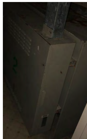
First floor elevator room.
