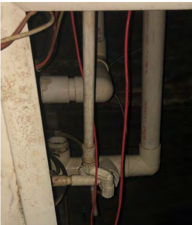
First floor management room pvc piping for indoor unit.
