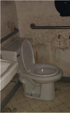
First floor public bathroom.
