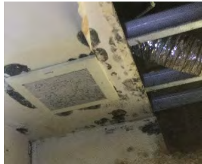
Exhaust vent and water damage to ceiling.
