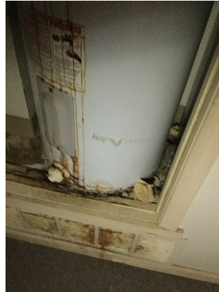
Hot water heater damaged.
