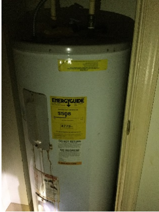
Connected hot water heater.
