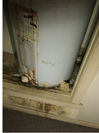
Hot water heater damaged.
