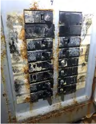
Damaged electrical panel.
