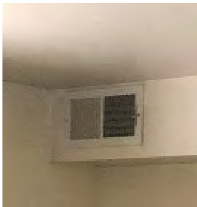
Typical vent in good shape
