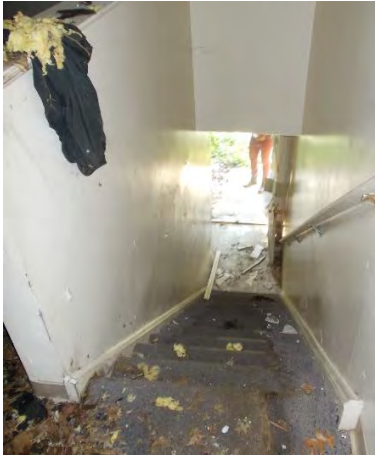
View looking down entry stairs to apartment entry door at grade.
