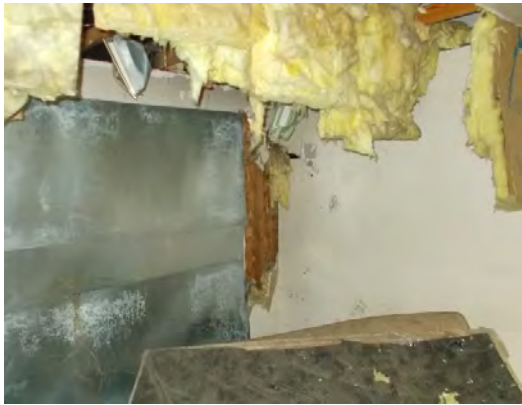
Detailed view of ceiling and exterior wall within bedroom.
