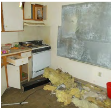
Depicts additional view of kitchen and rear windows facing rear yard.
