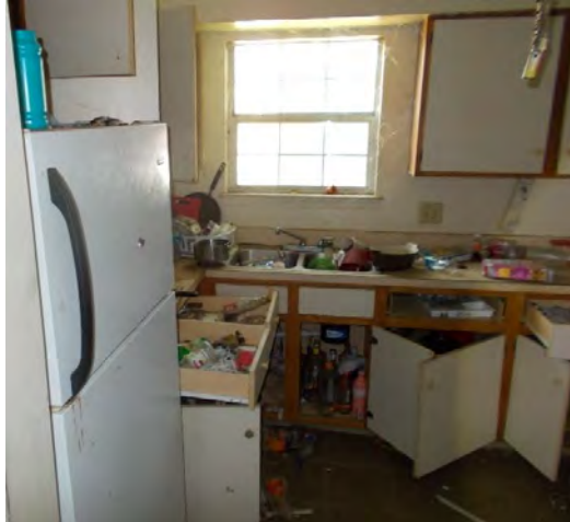
View of kitchen area adjacent to living room.
