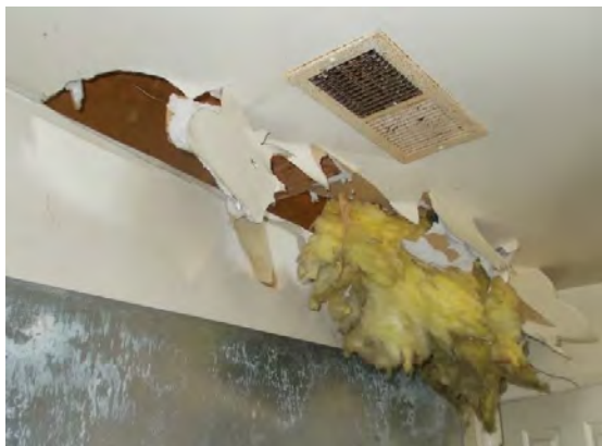
View of hallway closet beneath stairs to second floor.
