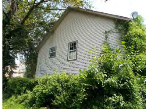
View of left side of building at unit 45 showing overgrown fencing along property line.
