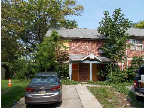
Exterior view of units 45 and 47.
