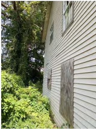
View looking West shows rear of buildings.
