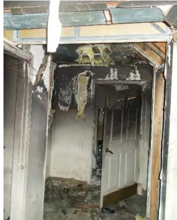
View looking at hallway to rear of apartment.
