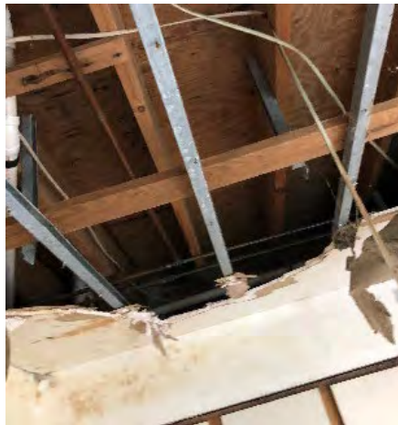
Damaged kitchen ceiling.
