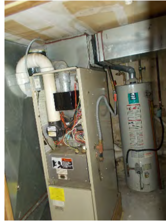
Hot water heater and furnace.
