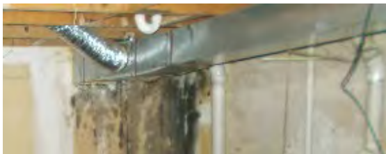
Duct damage.
