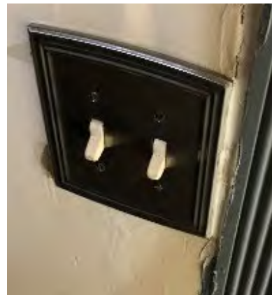
Light switch in good shape.
