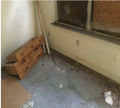
Hot water heater
