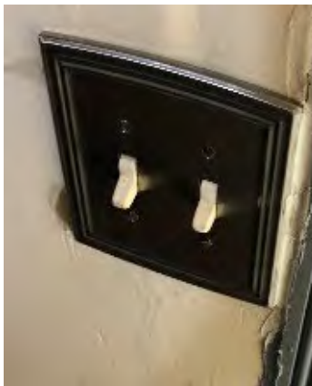
Light switch in good shape
