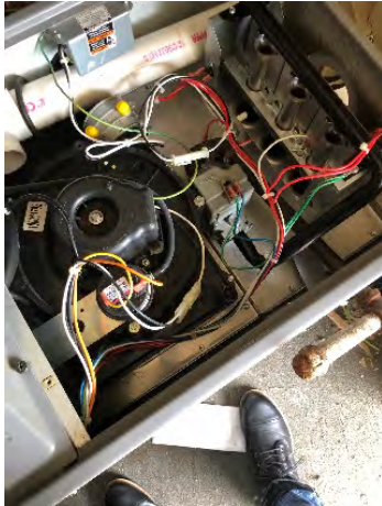
Another gas furnace disassembled and misplaced.
