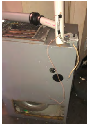
Gas furnace disassembled and misplaced.
