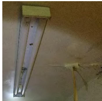
Kitchen light with water damage to ceiling.
