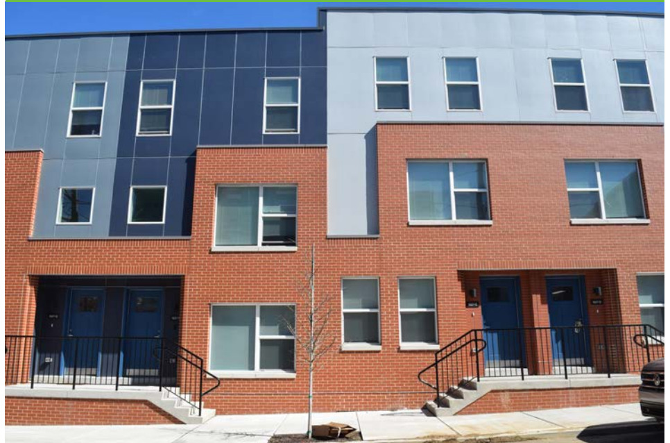
Sharswood Phase III, 1300 Block of N. 22nd Street.
