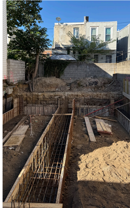
TKK homes under construction, 2317 Greenwich Street.
